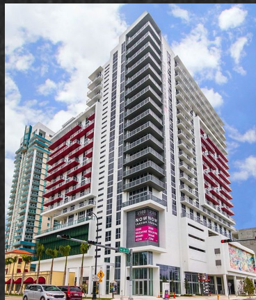
2500 BISCAYNE BLVD: $47M DEVELOPMENT; 2017 COMPLETION
