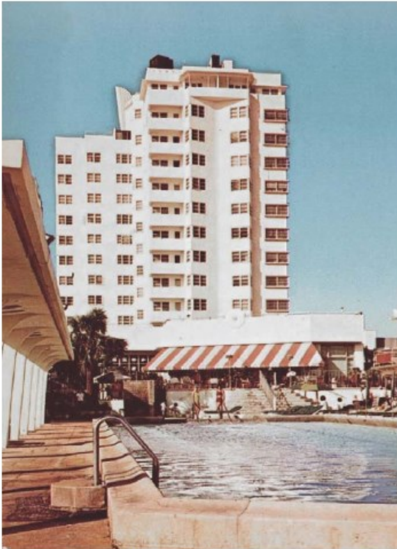
Striped awning at east elevation, c. 1950s
