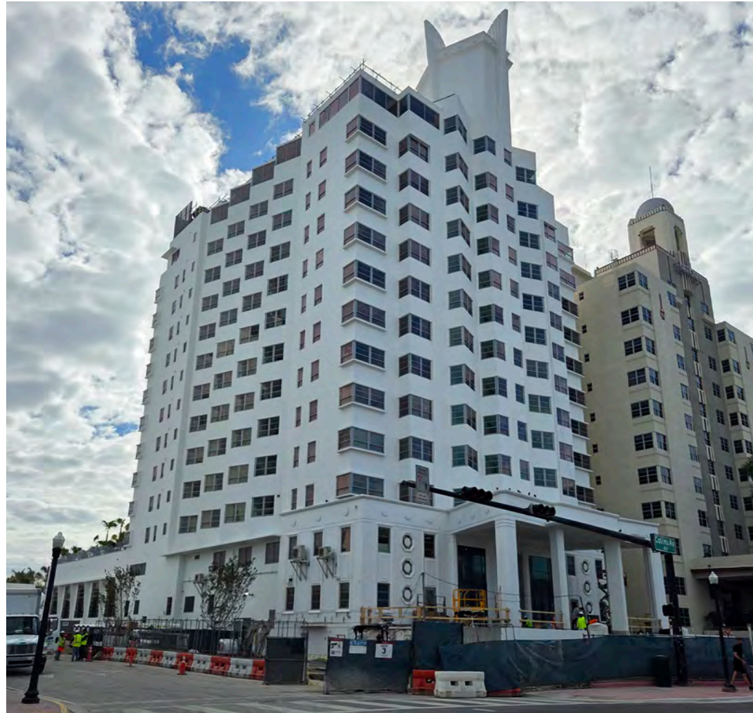
1. VIEW OF DELANO FACING SOUTH EAST
