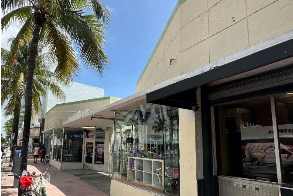
Figure 72. Detail of continuous concrete canopy, August 2023.
