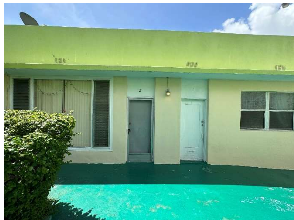
Figure 94. View of Unit 2, looking south, August 2023.
