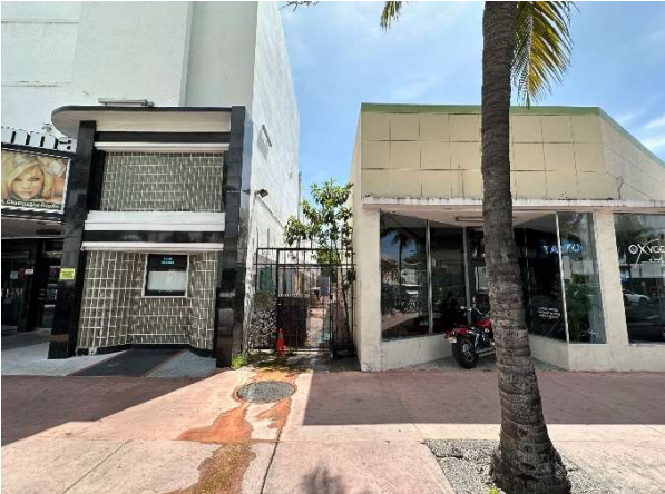
Figure 70. View of walkway north of 1515-1523 Washington Avenue, looking east, August 2023
