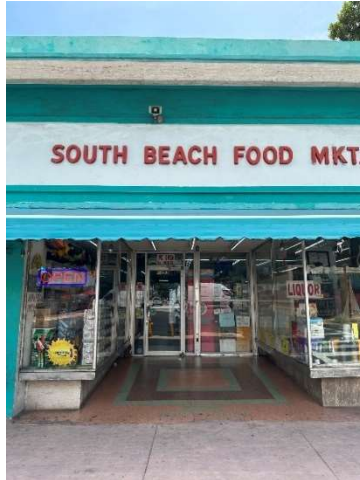
Figure 42. View of 1493 Washington Avenue, August 2023.
