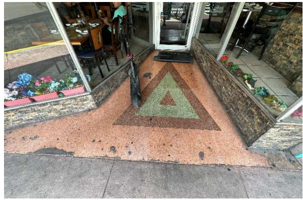
Figure 55. Detail of terrazzo floor at entrance to 1497 Washington Avenue, August 2023.
