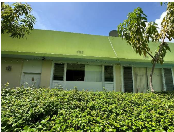
Figure 95. View of Unit 3, looking south, August 2023.
