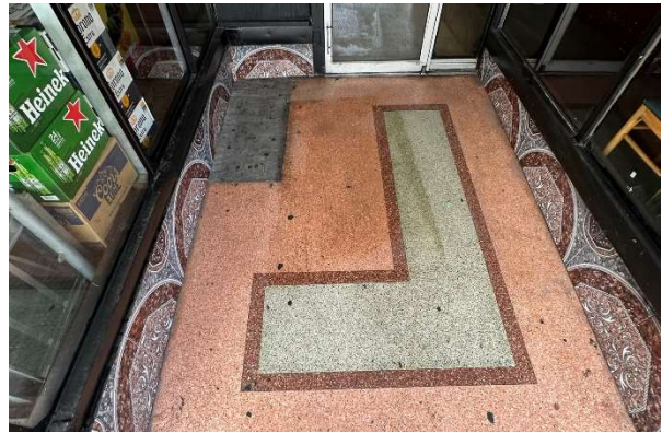
Figure 65. Detail of terrazzo floor at entrance to 1511 Washington Avenue, August 2023.
