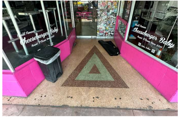
Figure 59. Detail of terrazzo floor at entrance to 1505 Washington Avenue, August 2023.
