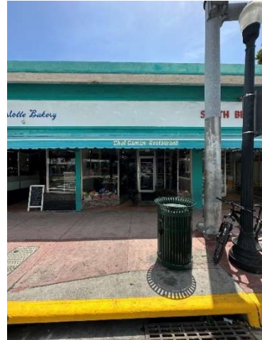
Figure 43. View of 1497 Washington Avenue, August 2023.
