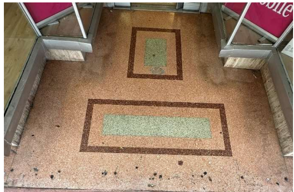
Figure 61. Detail of terrazzo floor at entrance to 1507 Washington Avenue, August 2023.
