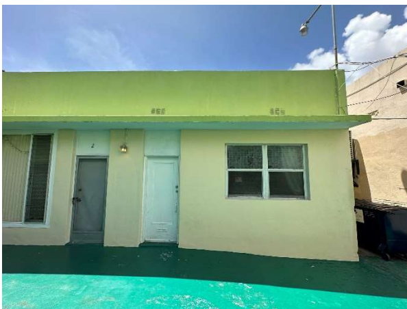
Figure 93. View of Unit 1, looking south, August 2023.
