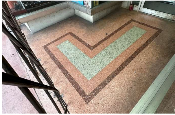
Figure 63. Detail of terrazzo floor at entrance to 1509 Washington Avenue, August 2023.
