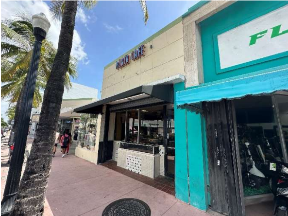
Figure 69. Detail of connection of the buildings at 1491-1513 and 1515-1523 Washington Avenue, August 2023
