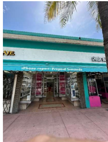
Figure 46. View of 1507 Washington Avenue, August 2023.
