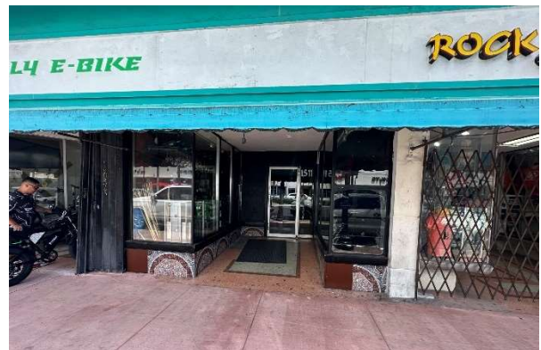
Figure 40. Detail of continuous signboard and awning, August 2023.
