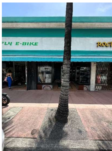
Figure 48. View of 1511 Washington Avenue, August 2023.
