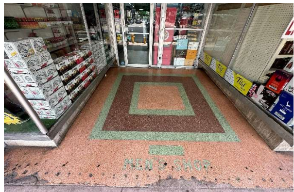
Figure 53. Detail of terrazzo floor at entrance to 1493 Washington Avenue, August 2023.
