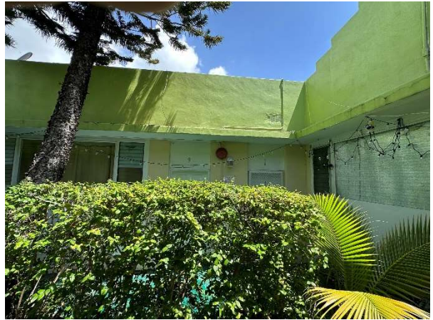
Figure 100. View of Units 8 and 9, looking northeast, August 2023.
