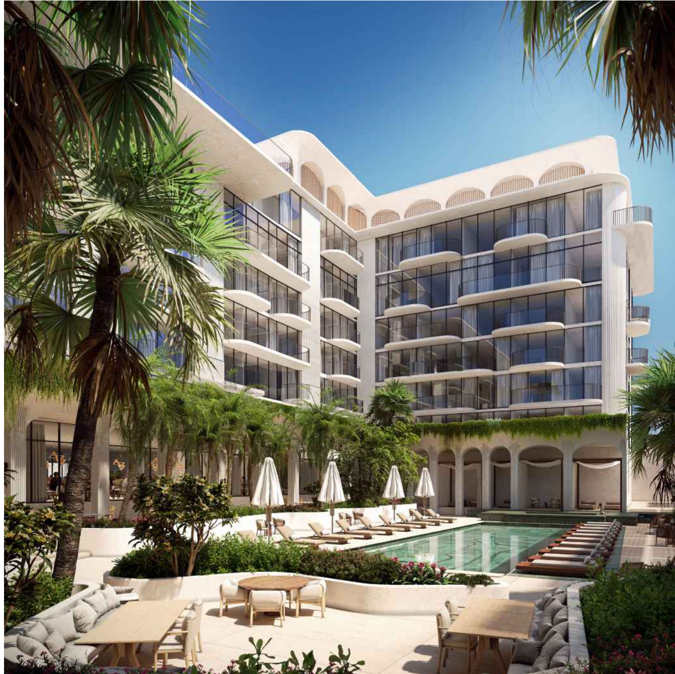
NORTHWEST FACADE OF INNER POOL COURTYARD
