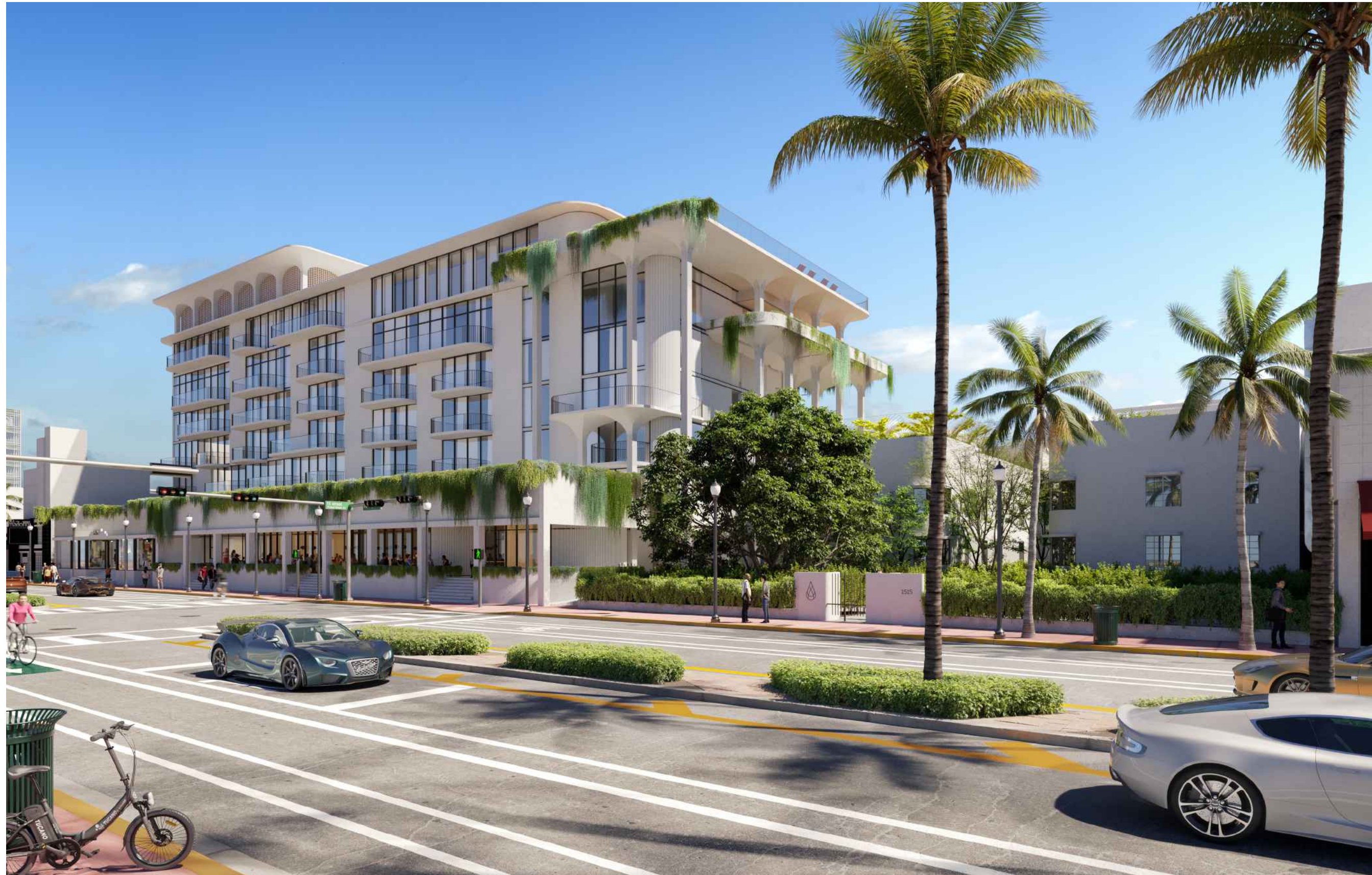
WEST FACADE OF PROPERTY, VIEW OF WASHINGTON ENTRANCE
