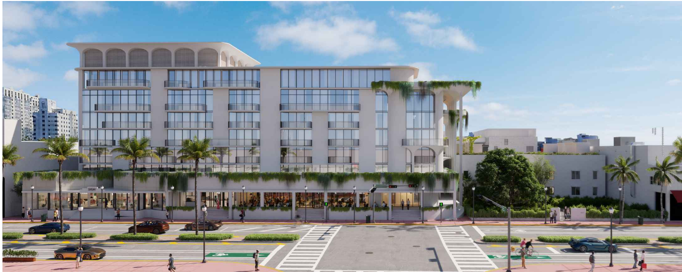
WEST FACADE OF PROPERTY, VIEW OF WASHINGTON ENTRANCE
