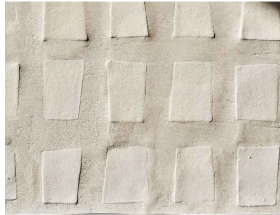
F. DECORATIVE TILE @ VAULTED CEILINGS OF RESTURANT
