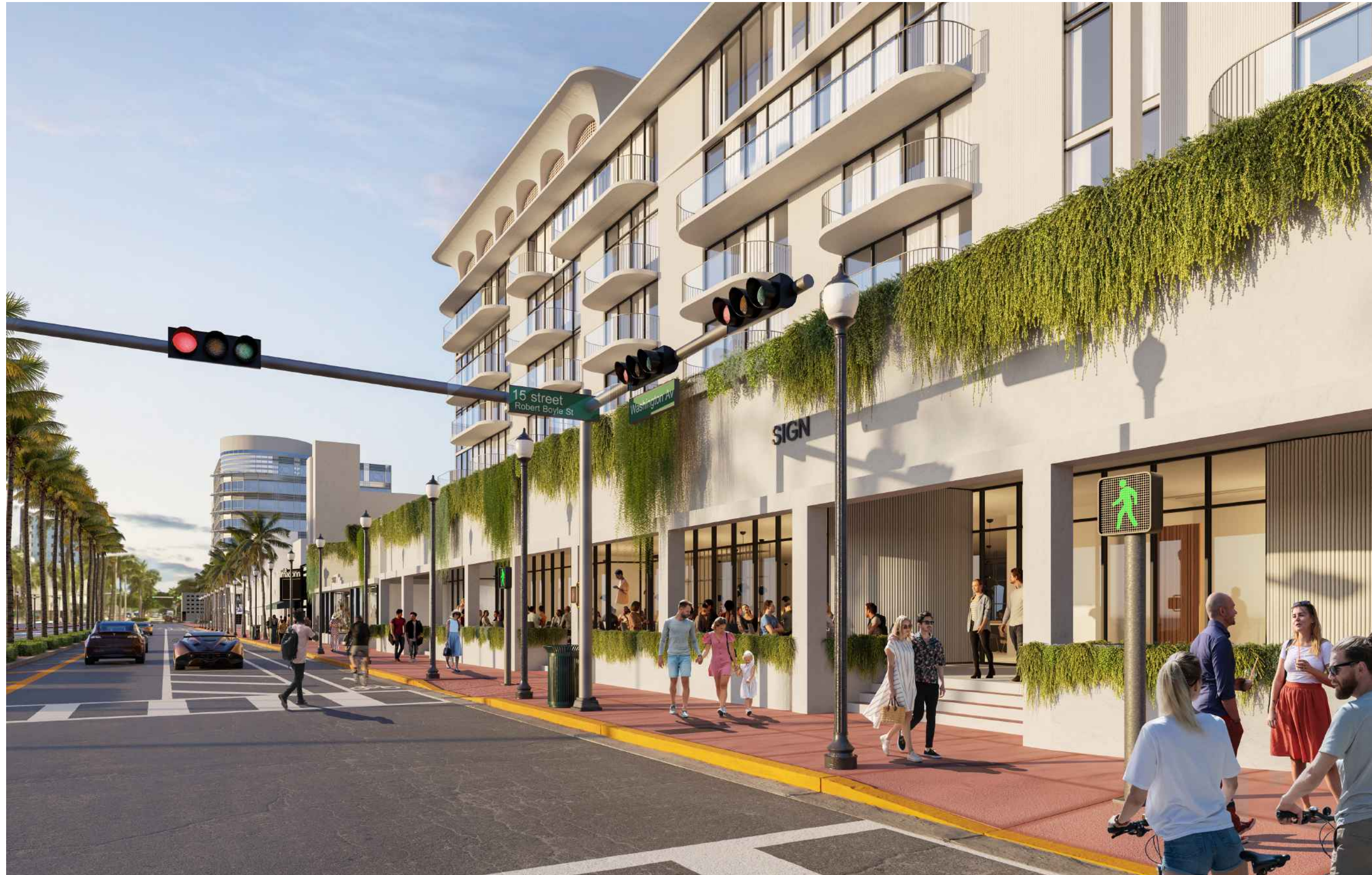
WEST FACADE OF PROPERTY, VIEW OF FUTURE C.O.R.
