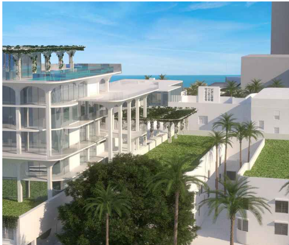
VIEW OF BUILDING CONNECTION POINTS FROM THE WEST
