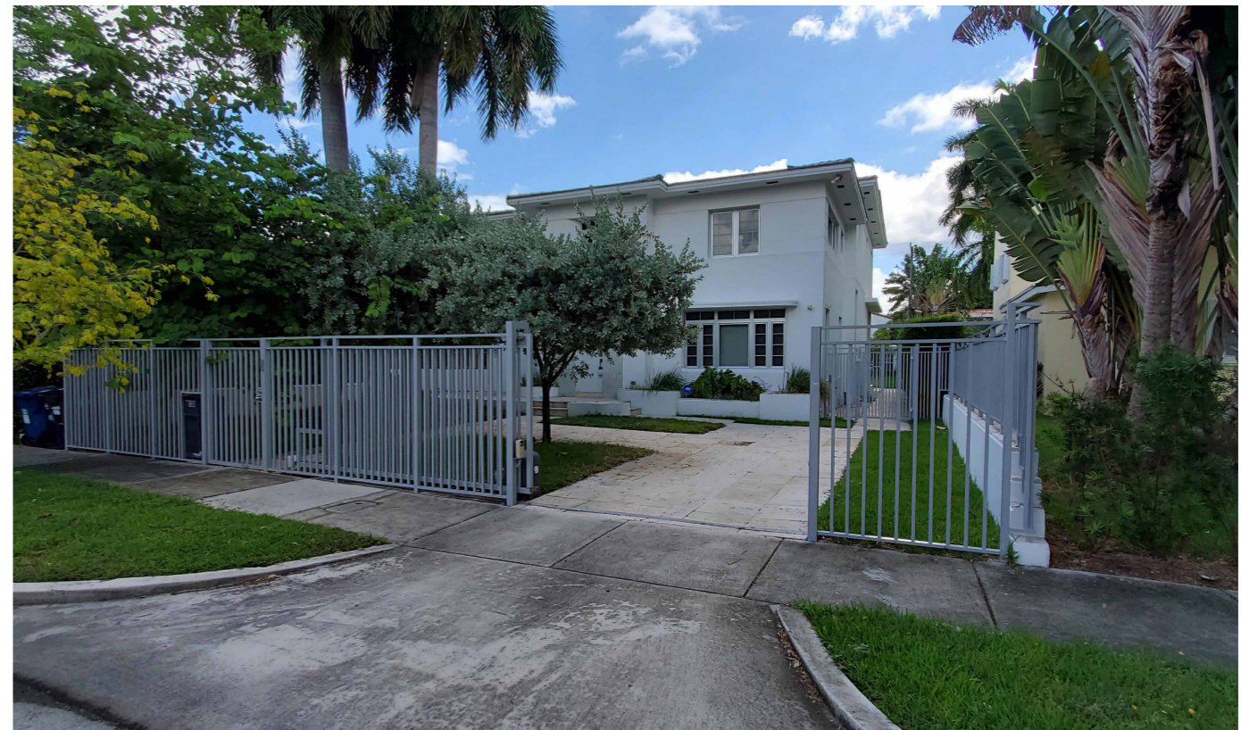
16 VIEW OF LOT 1815 FACING EAST.
