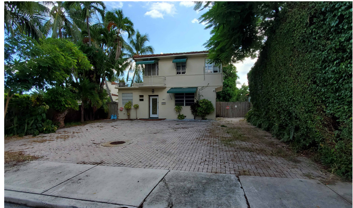
14 VIEW OF LOT 1827 FACING EAST.
