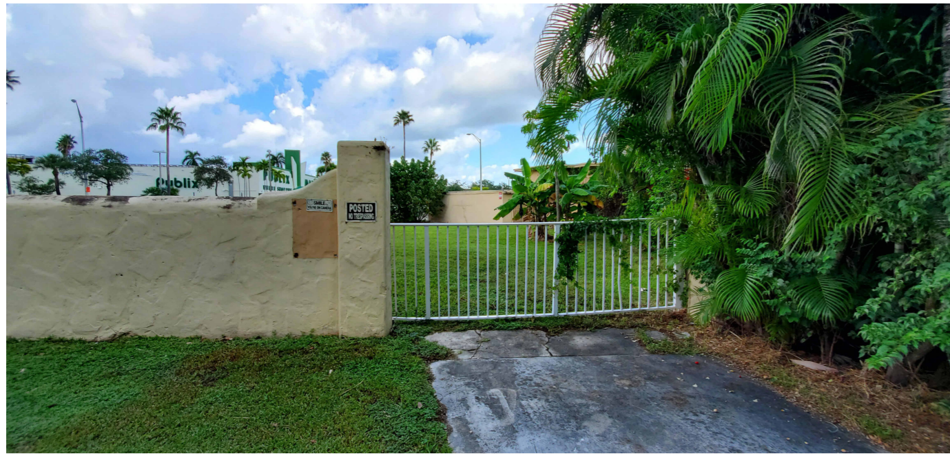
13 VIEW OF LOT 4 FROM 18TH STREET BEFORE DEMOLITION OF 1818 MICHIGAN AVE (LOT 3) 1 1/2" = 1'-0"
