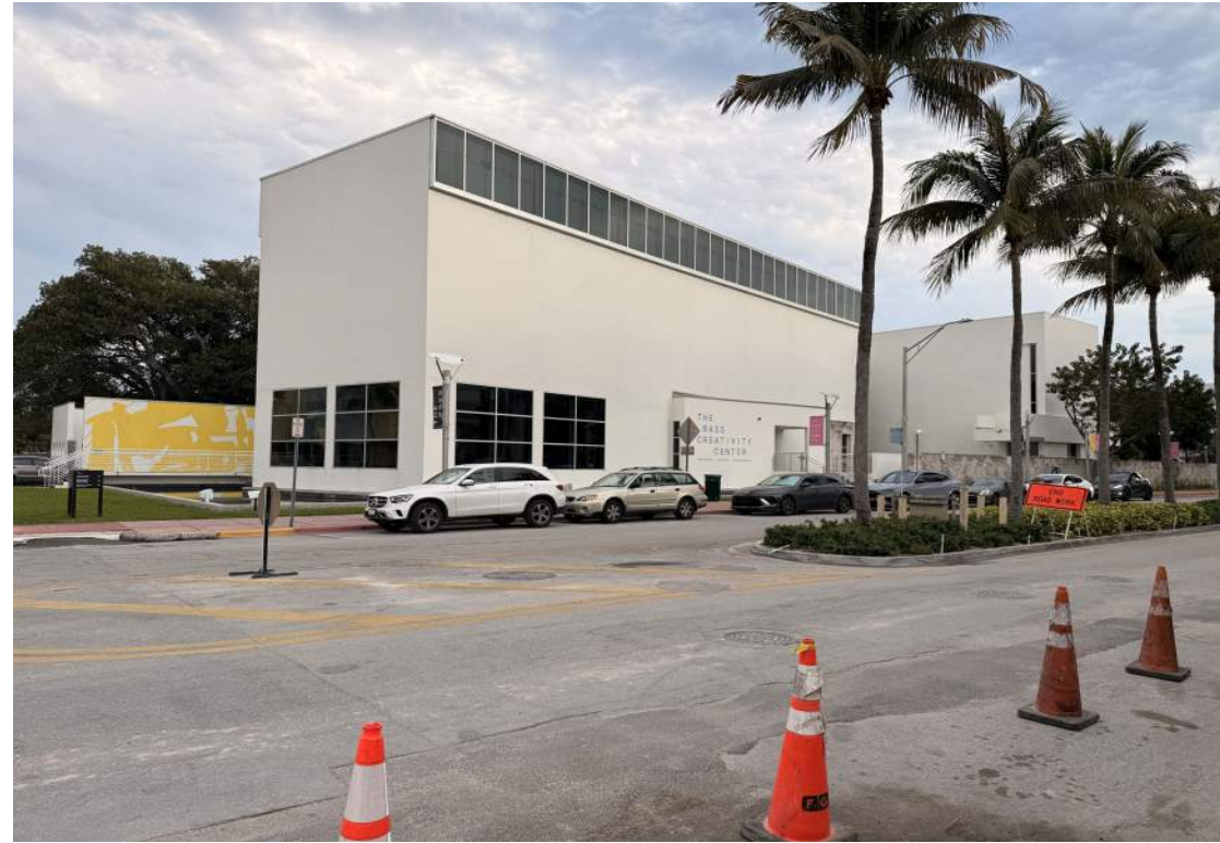
1 - VIEW FROM PARK AVENUE AND 22ND ST CORNER TOWARD THE EXISTING BUILDING, 2026.02.11
