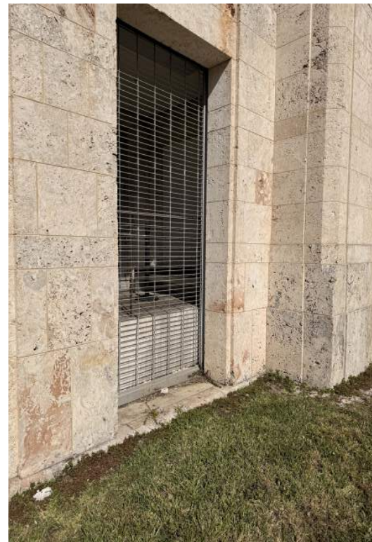
4 - EXISTING LOGGIA OPENINGS, 2026.02.11
