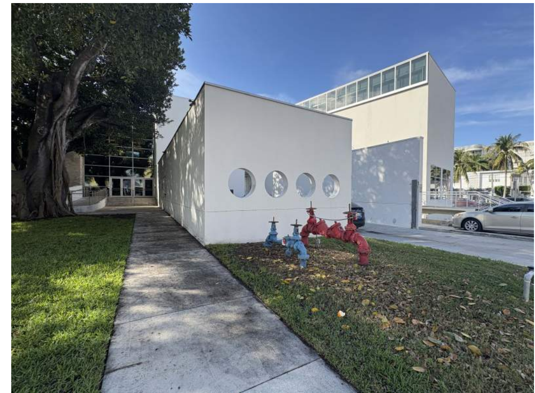
12 - VIEW FROM 22ND ST TOWARD THE EXISTING BUILDING, 2026.02.11
