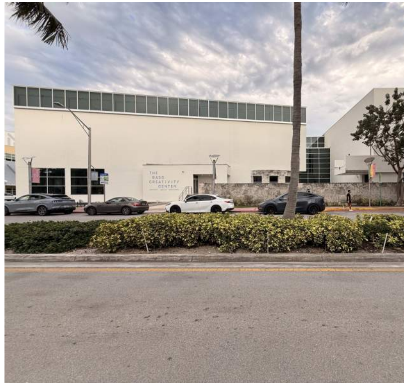
2 - VIEW ALONG PARK AVENUE TOWARD THE EXISTING BUILDING, 2026.02.11
