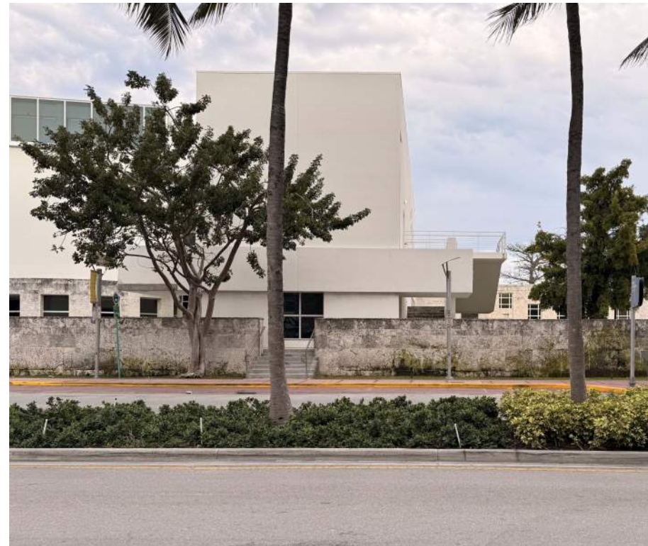
3 - VIEW ALONG PARK AVENUE TOWARD THE EXISTING BUILDING, 2026.02.11
