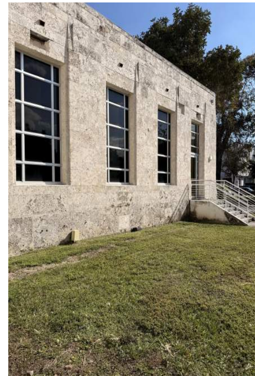
6 - EXTERIOR EXISTING STAIRS, 2026.02.11
