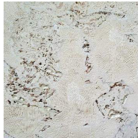
EXTERIOR SITE WALL FLORIDA KEYSTONE
