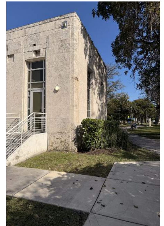
7 - SOUTH EXISTING BUILDING CORNER, 2026.02.11
