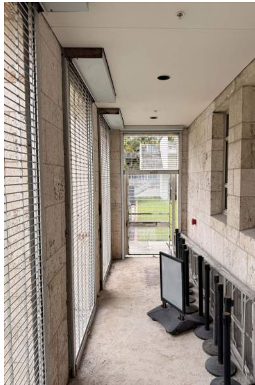
INTERIOR VIEW OF (S) LOGGIA, 2026.04.07
