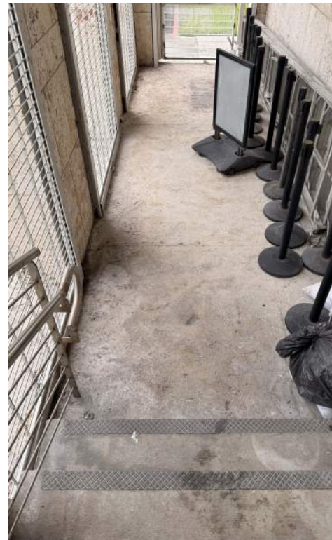
INTERIOR VIEW OF (S) LOGGIA, 2026.04.07
