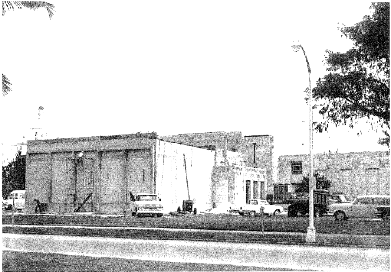
WESTERN WING OF BASS MUSEUM UNDER CONSTRUCTION 1965 courtesy CITY OF MIAMI BEACH PHOTO ARCHIVES
