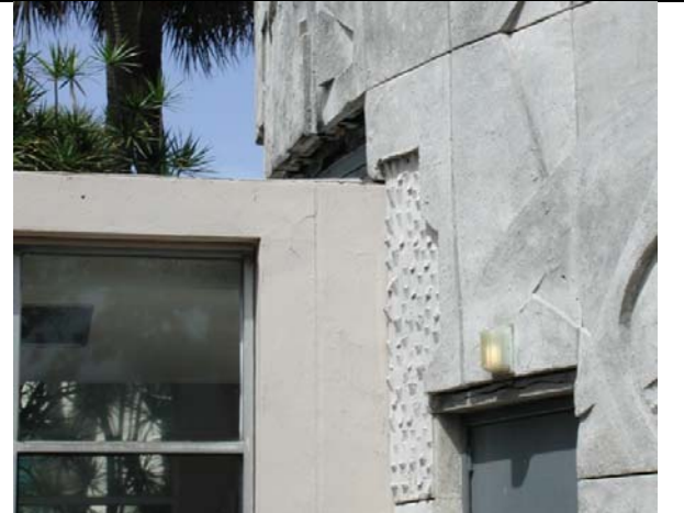
2004 - Rotunda bridge detail
