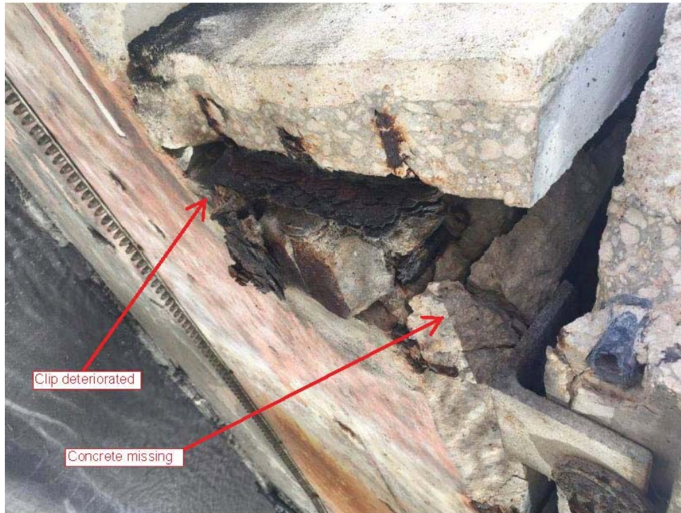
2022 Photo of south window wall condition at underside of panels:
