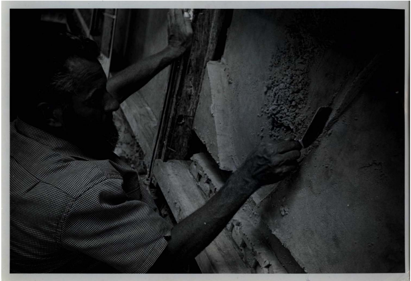
Albert Vrana carving sand molds for the Rotunda:
