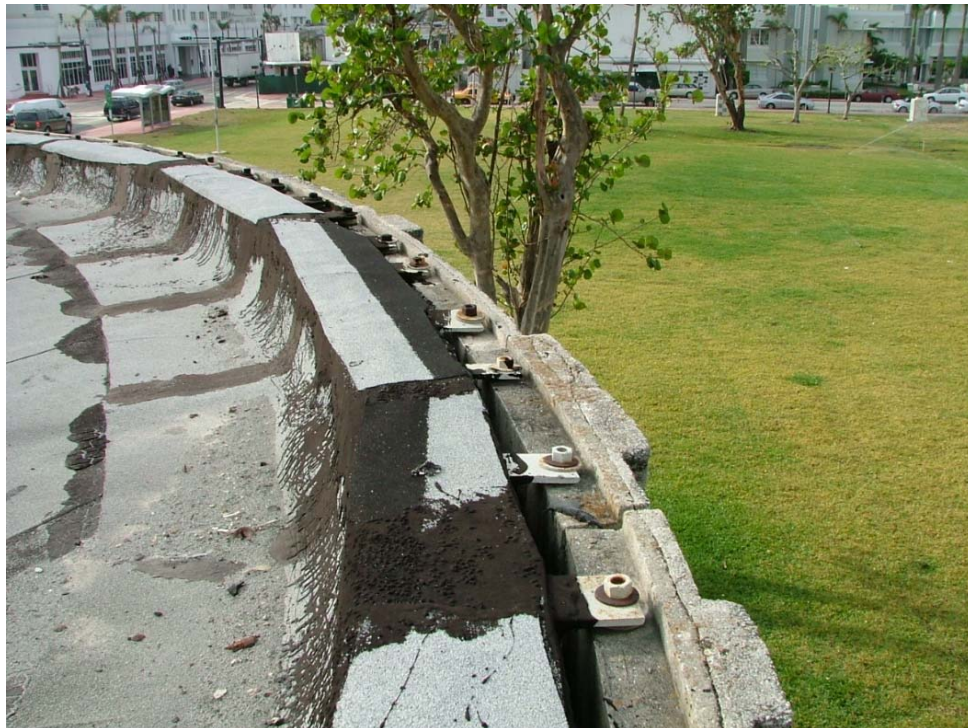
2006 photo of roof showing panels connection:
