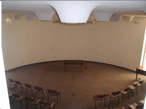
2004 – Rotunda Interior – Ceiling Detail
