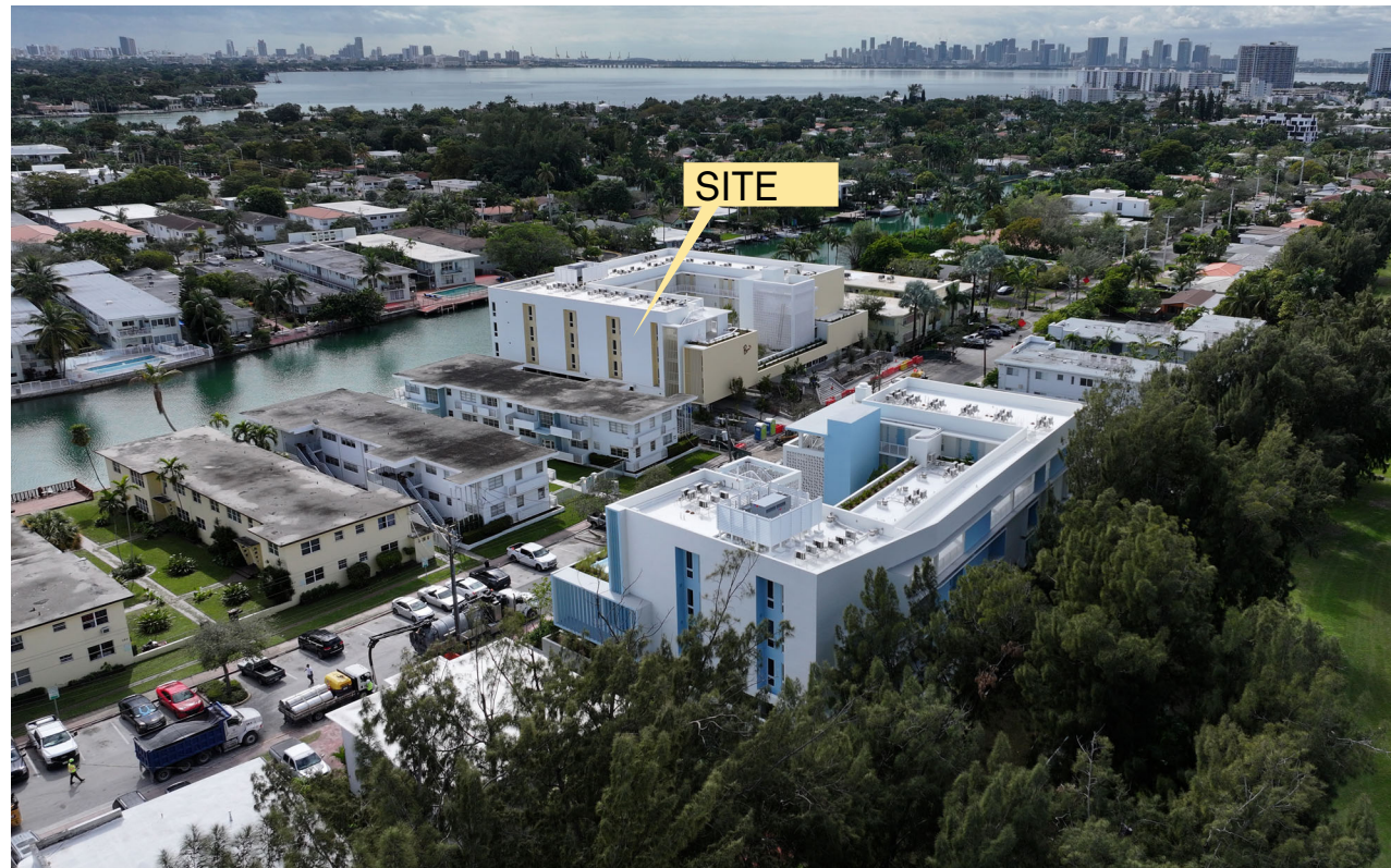
AERIAL VIEW / FROM NORTHEAST
