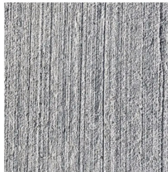
FINISH: CONCRETE LIGHT BROOM FINISH COLOR: GRAY
