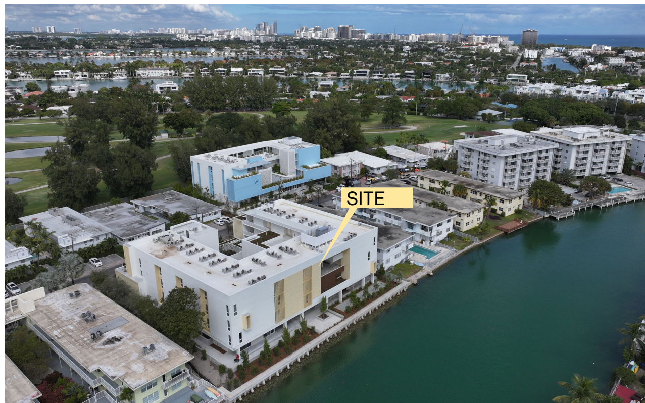
AERIAL VIEW / FROM SOUTHWEST
