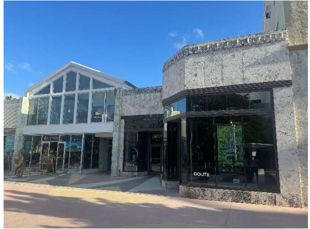
Figure 16. Detail of central bay and west wing at 918-932 Lincoln Road, April 2026.
