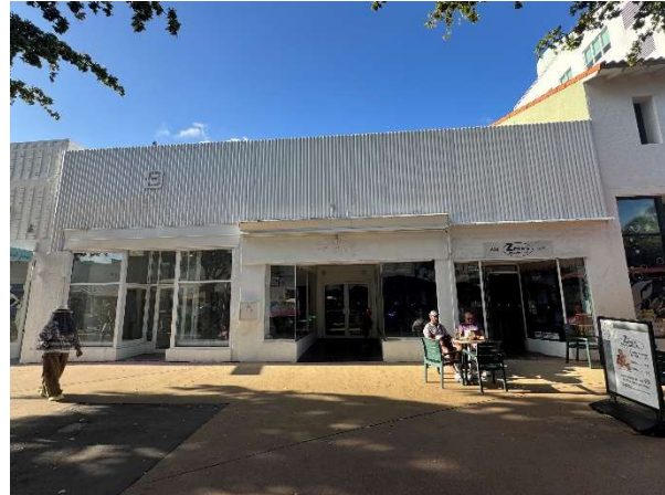
Figure 6. 625-631 Lincoln Road, April 2026.
