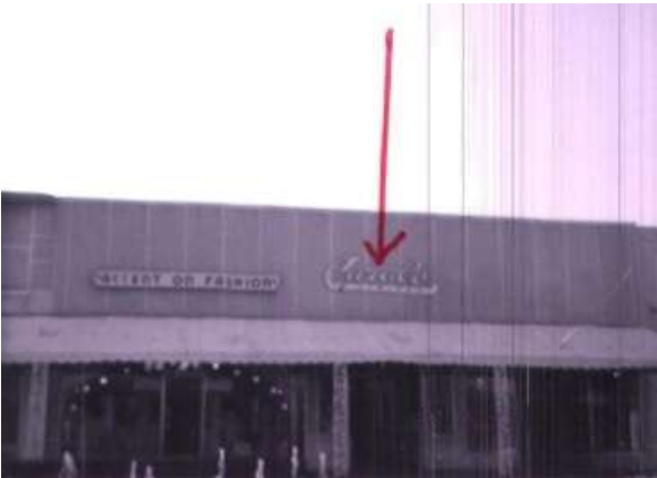
Figure 32. View of upper façade showing absence of vertical piers, 1971. (Miami-Dade County Property Assessor)
