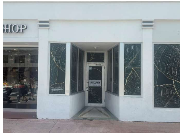
Figure 20. Detail of 718 Lincoln Road, March 2026.
