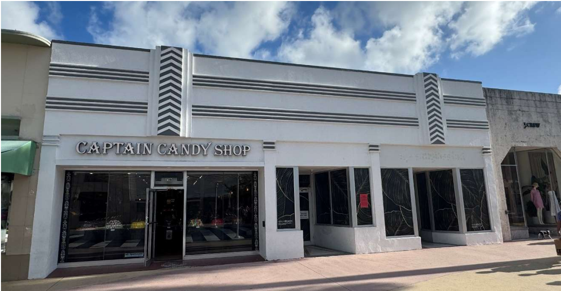
Figure 17. 716-720 Lincoln Road, April 2026.
