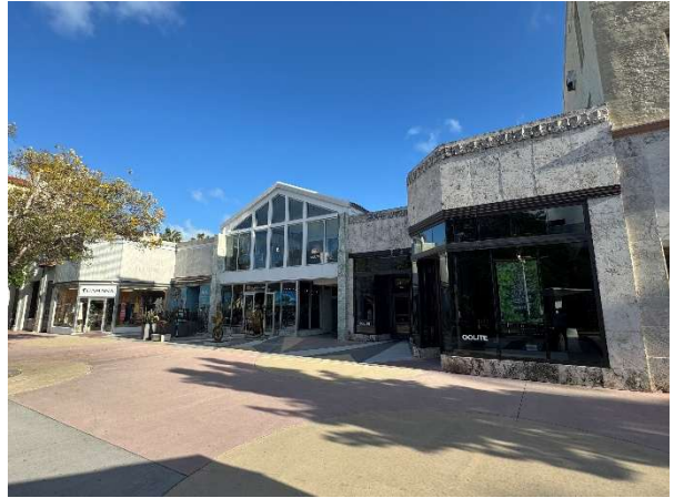
Figure 14. 918-932 Lincoln Road, April 2026.
