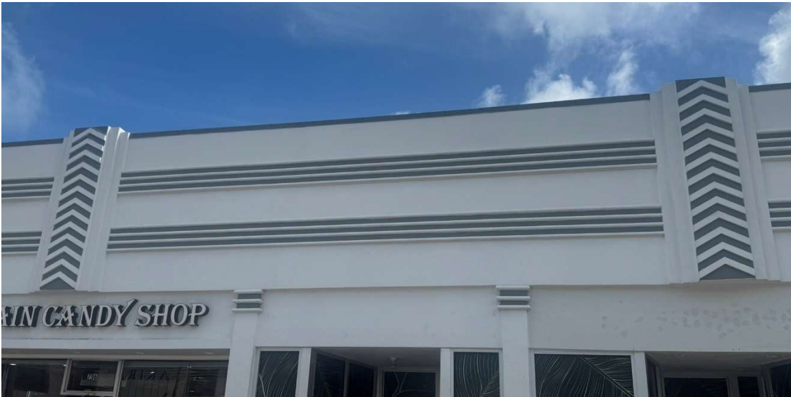
Figure 18. Detail of upper façade at 716-720 Lincoln Road, March 2026.
