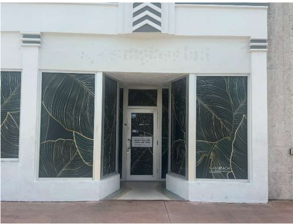
Figure 21. Detail of 720 Lincoln Road, March 2026.
