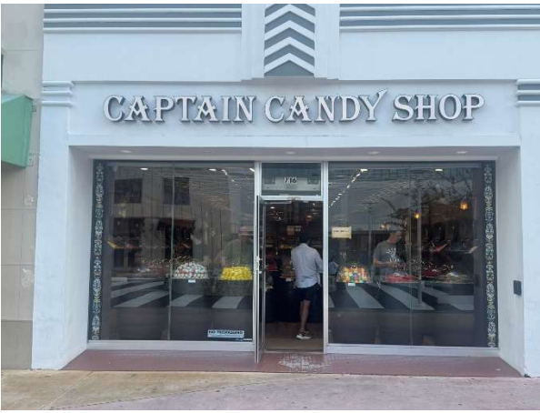
Figure 19. Detail of 716 Lincoln Road, March 2026.
