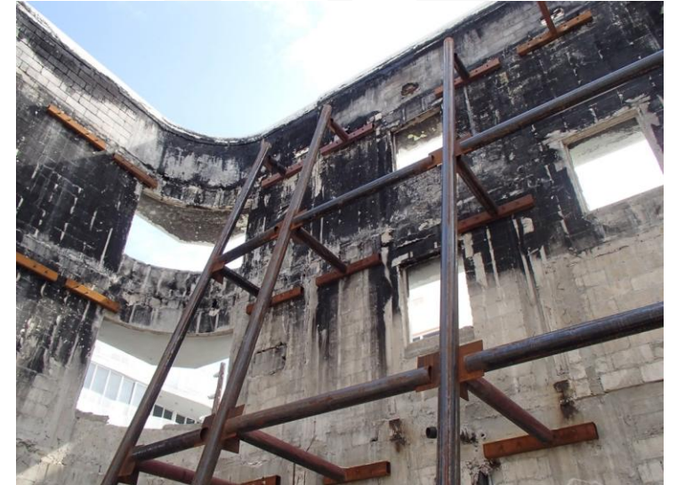
Collins Park Bracing
