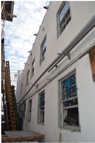
Figure 44. View of North Elevation, looking southeast, November 2025.
