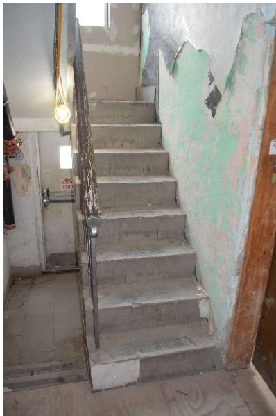
Figure 66. View of rear stairs, looking east, November 2025.
