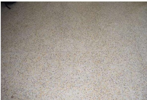
Figure 58. Detail of original terrazzo flooring, November 2025.
