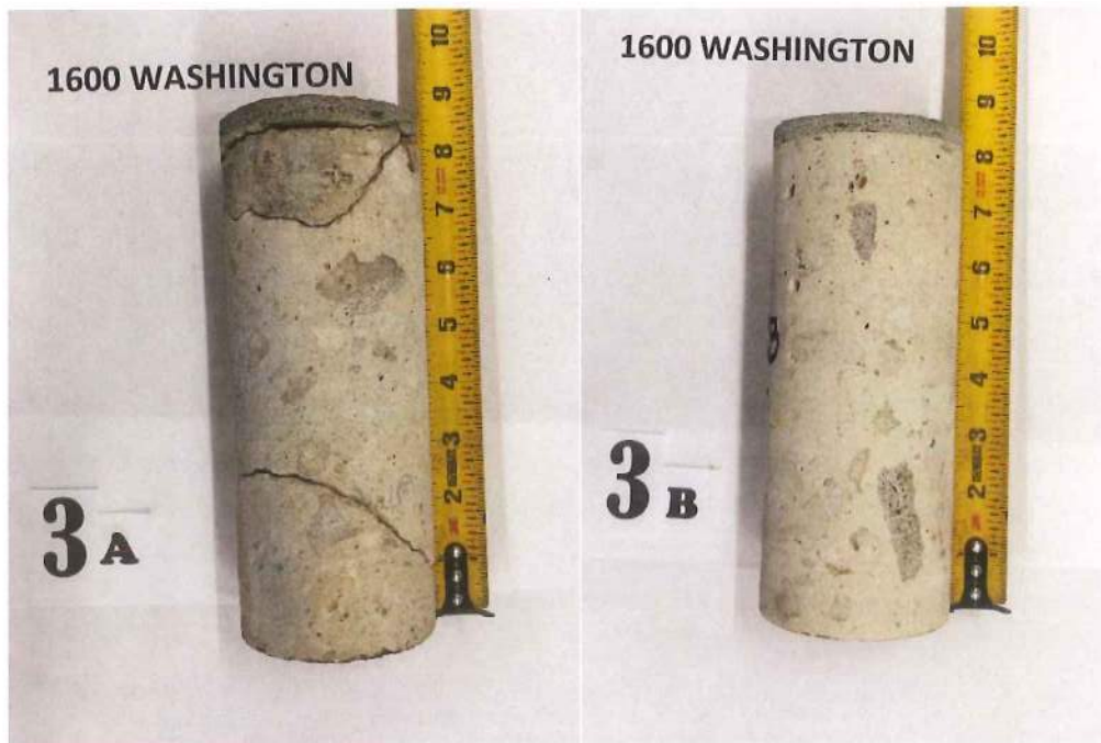
Figure 4: Photograph of Core Samples Level 1 (Compression/Chloride/Carbonation Samples)
