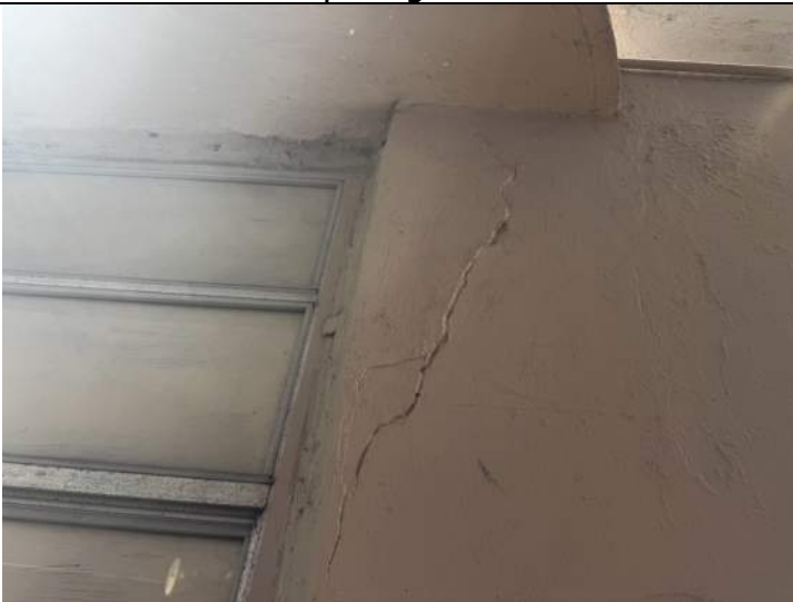
Concrete cracking
