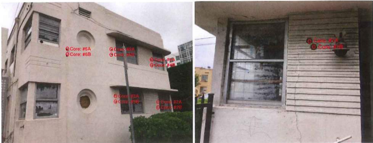
Figure 1: 1600 Washington Ave. - Approximate Concrete Core Locations
