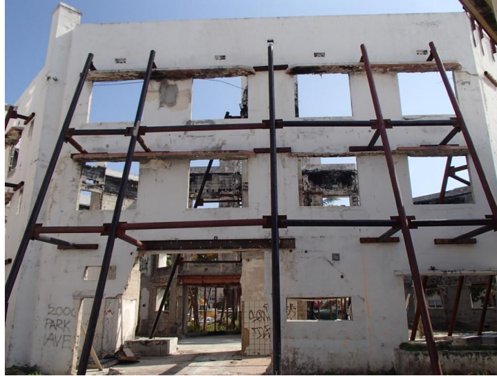
Collins Park Bracing
