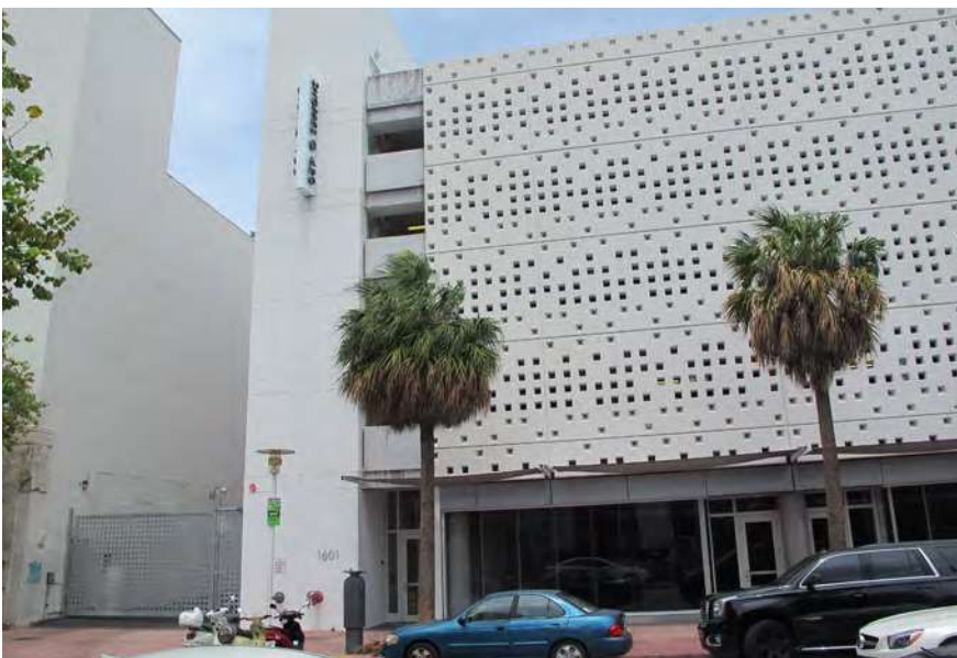
Drexel Avenue Lobby entrance to 420 Garage
