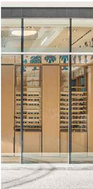
'STICK' STOREFRONT SYSTEMS OVER CLEAR ANODIZED ALUMINUM FOR RETAIL AND RESIDENTIAL LOBBY
