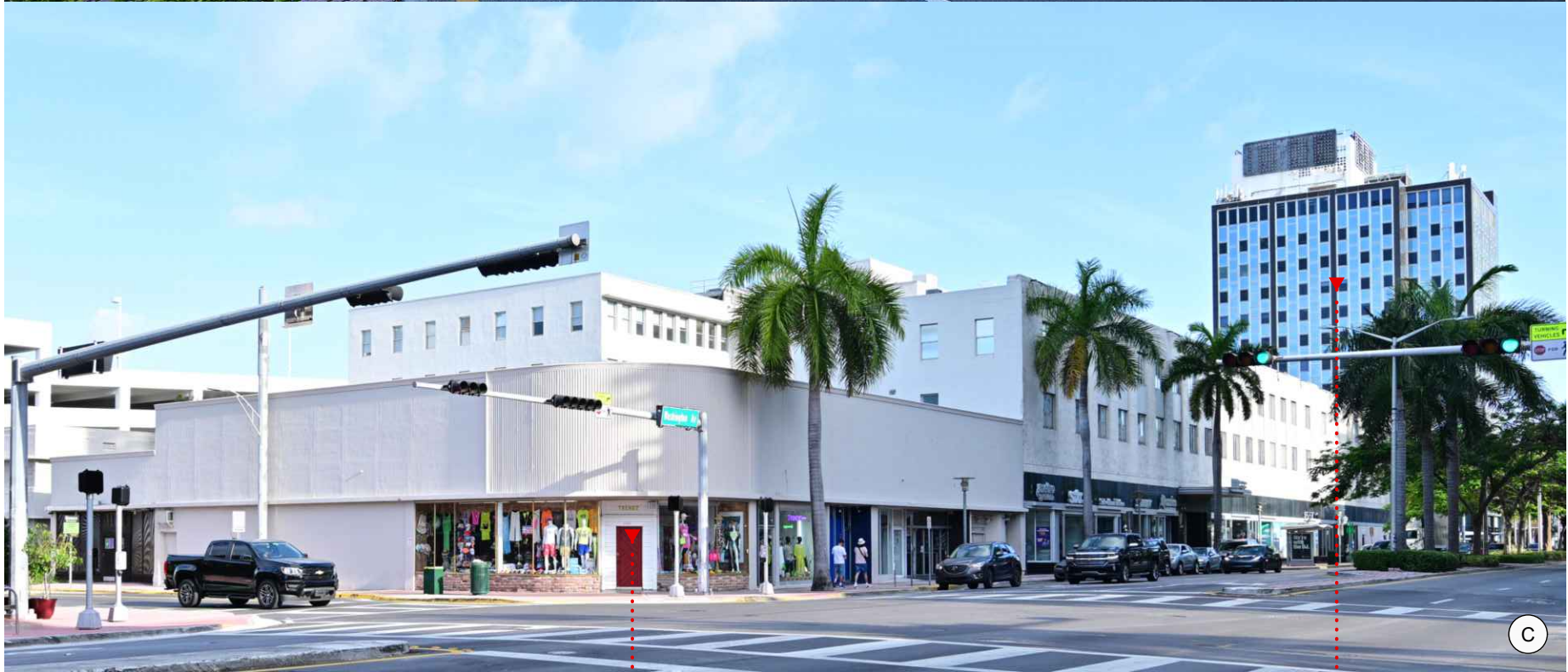
1600 WASHINGTON AVE EXISTING BUILDING TO BE DEMOLISHED
