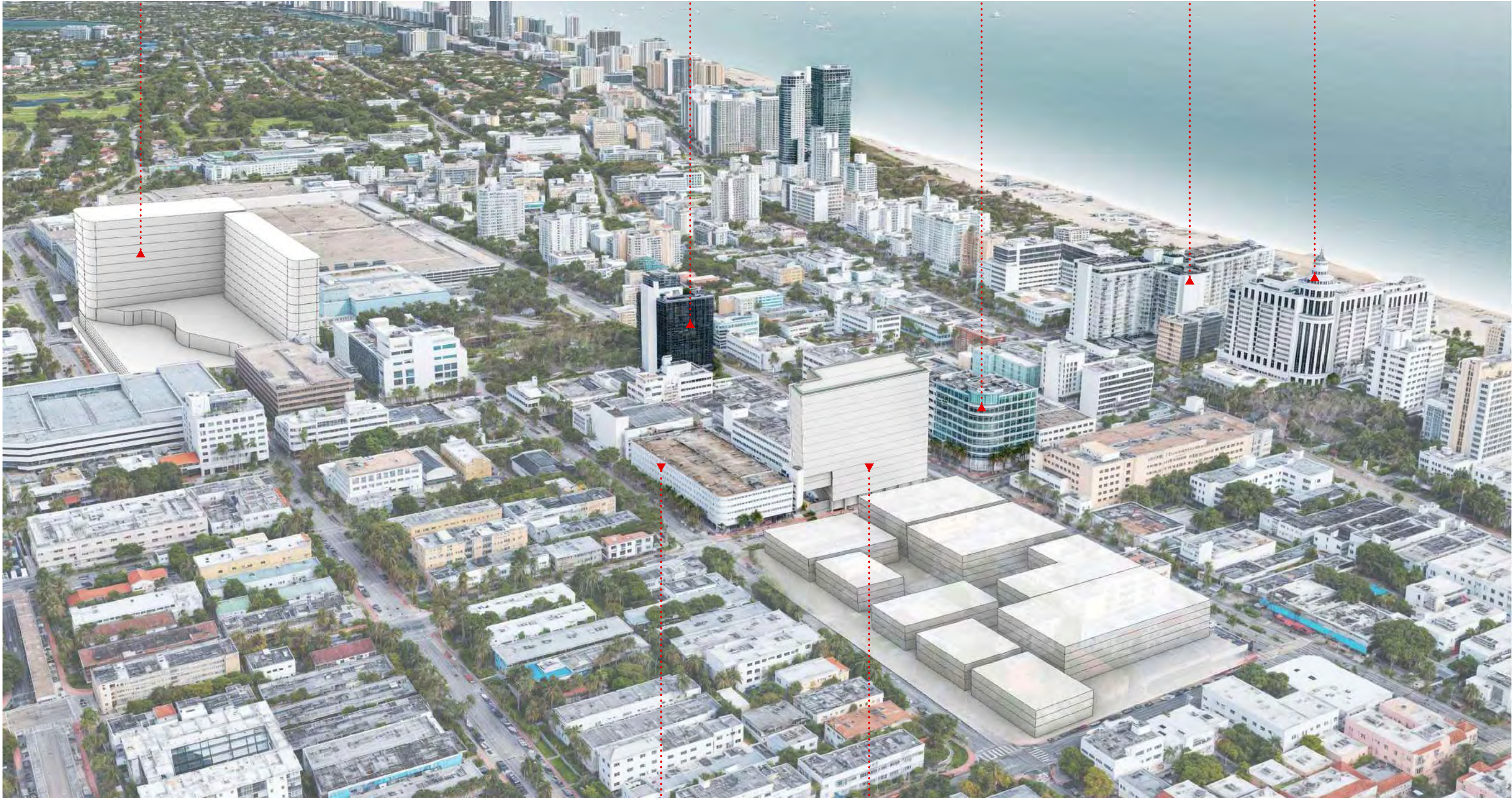
1601 DREXEL AVE EXISTING GARAGE BUILDING TO REMAIN
