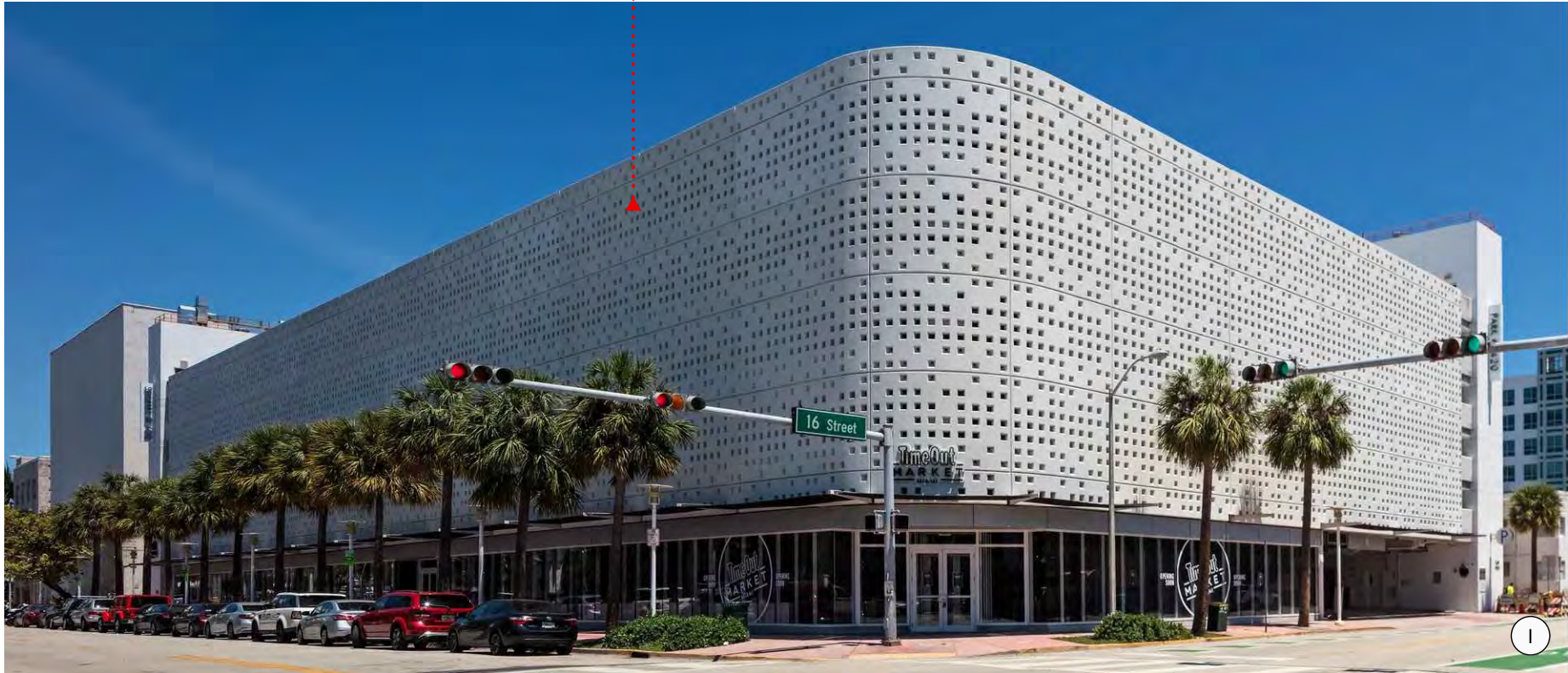
1601 DREXEL AVE EXISTING GARAGE BUILDING TO REMAIN
