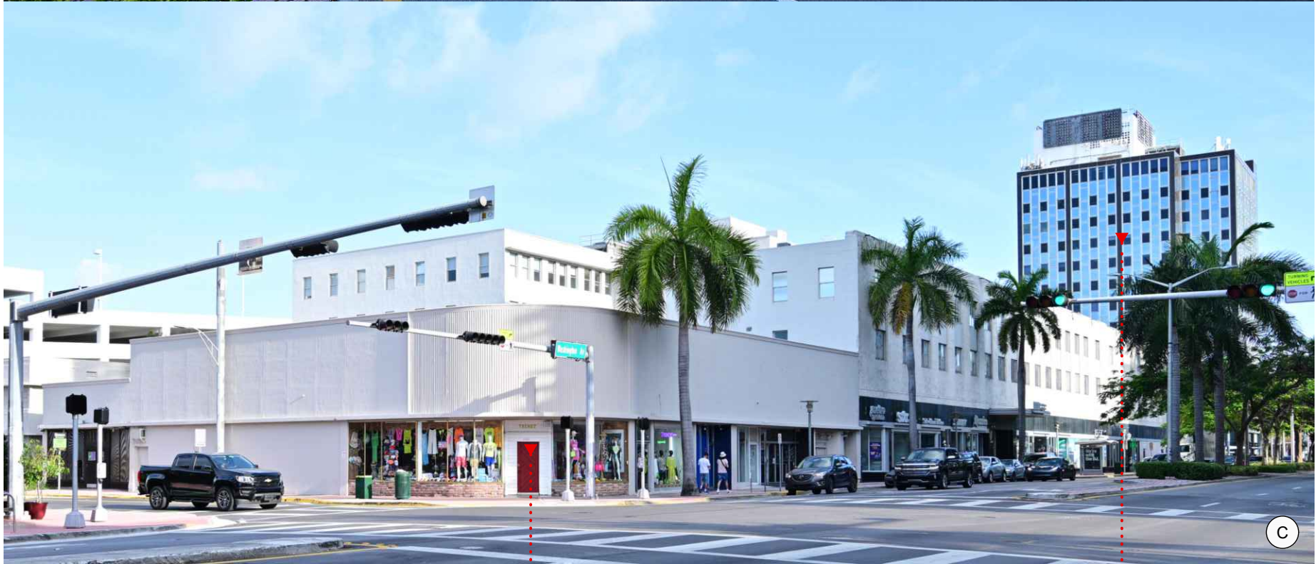
1600 WASHINGTON AVE EXISTING BUILDING TO BE DEMOLISHED
