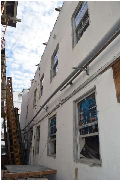
Figure 44. View of North Elevation, looking southeast, November 2025.
