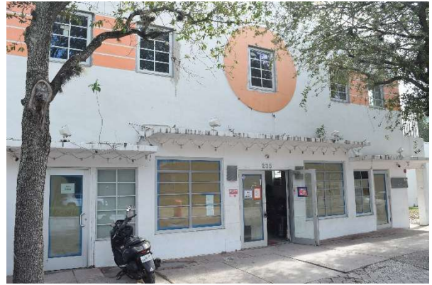
Figure 41. Detail of fenestration at Front Façade, November 2025.
