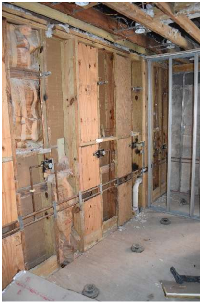
Figure 72. Detail of partially completed bathroom, November 2025.
