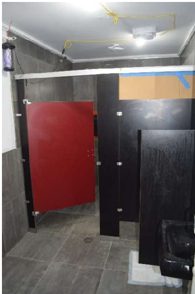
Figure 62. View of Men's Room, looking north, November 2025.
