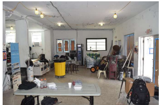
Figure 51. View of former Lobby, looking south, November 2025.
