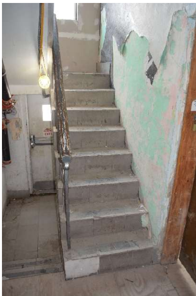
Figure 66. View of rear stairs, looking east, November 2025.
