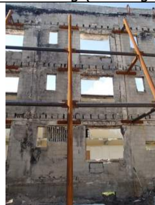
Collins Park bracing
