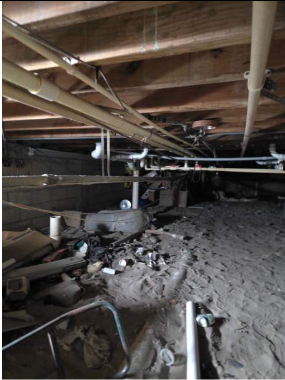
Crawl space under first floor
