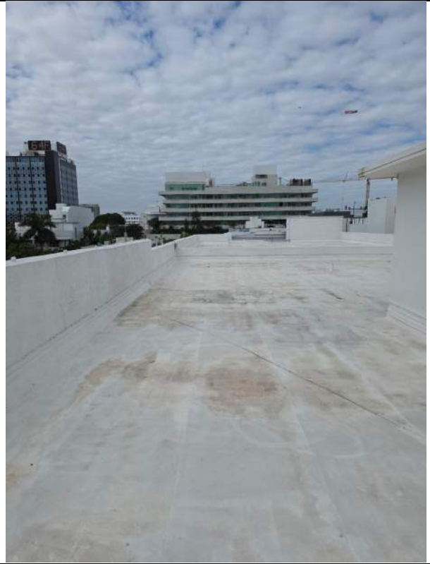
Roof view looking West
