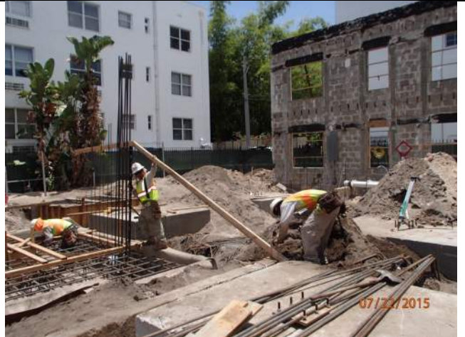
Ansonia bracing (in background)
