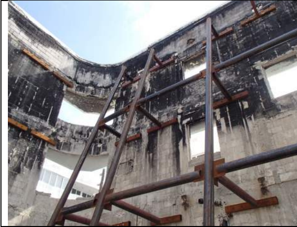
Collins Park bracing
