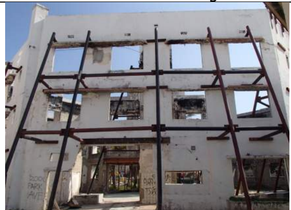
Collins Park bracing
