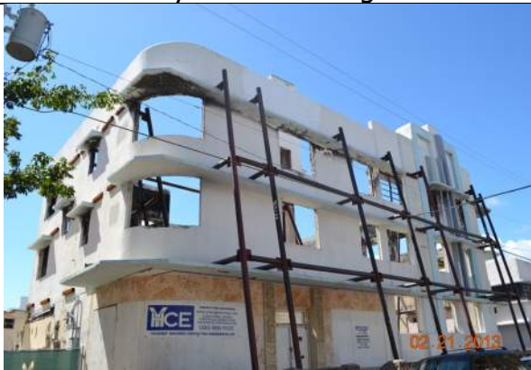
Collins Park bracing
