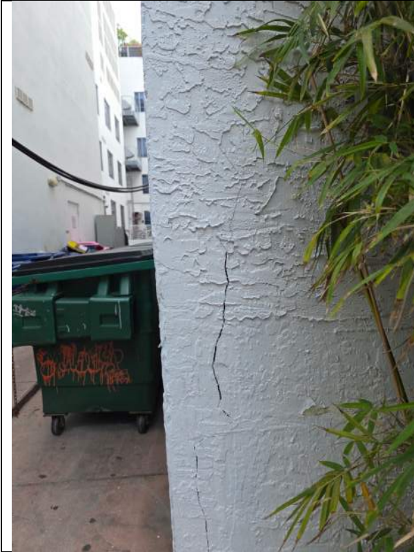
Concrete restoration of corner columns
