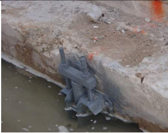
Carlton foundations improvements
