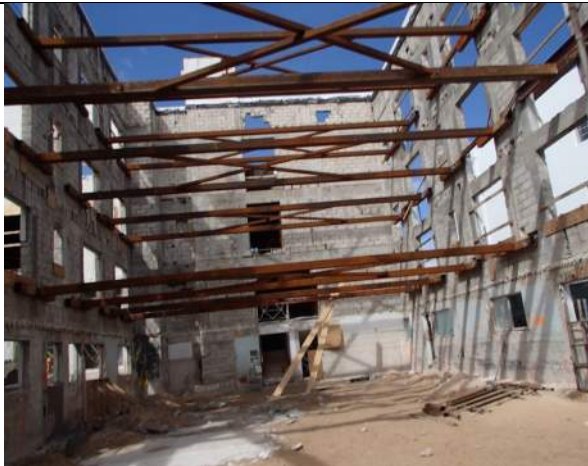
Carlton Hotel Interior bracing
