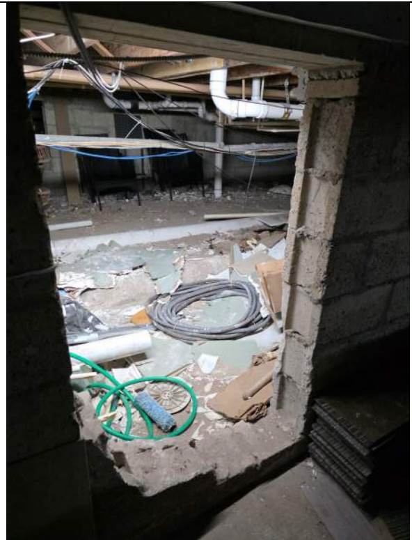
Crawl space under first floor
