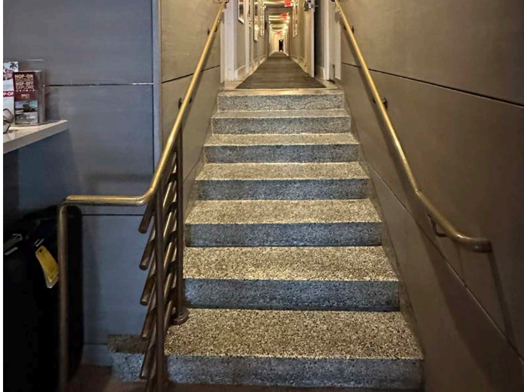
Ground floor - terrazzo stairs to corridor
