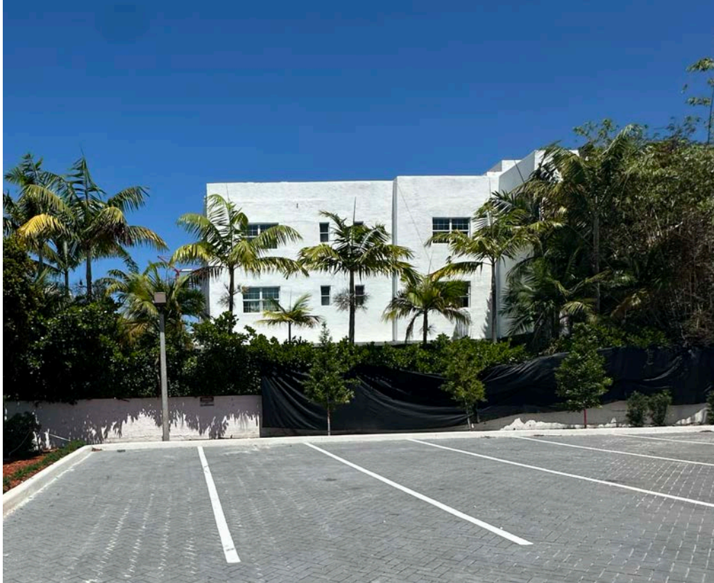
South facade viewed from adjacent parking lot
