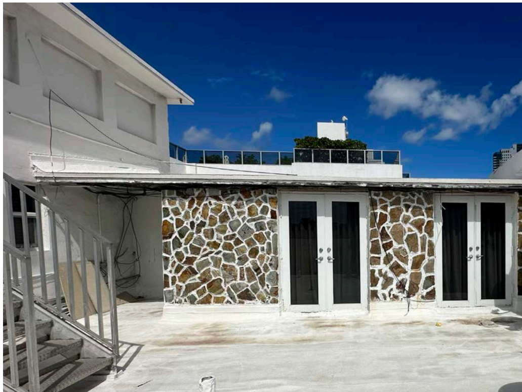
Roof level - penthouse
