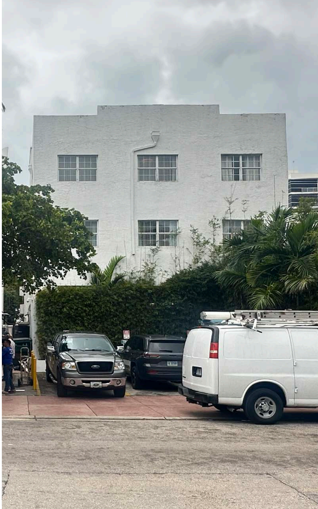
James Avenue facade
