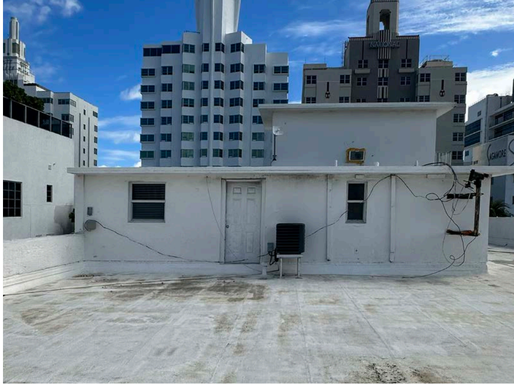
Roof level - penthouse
