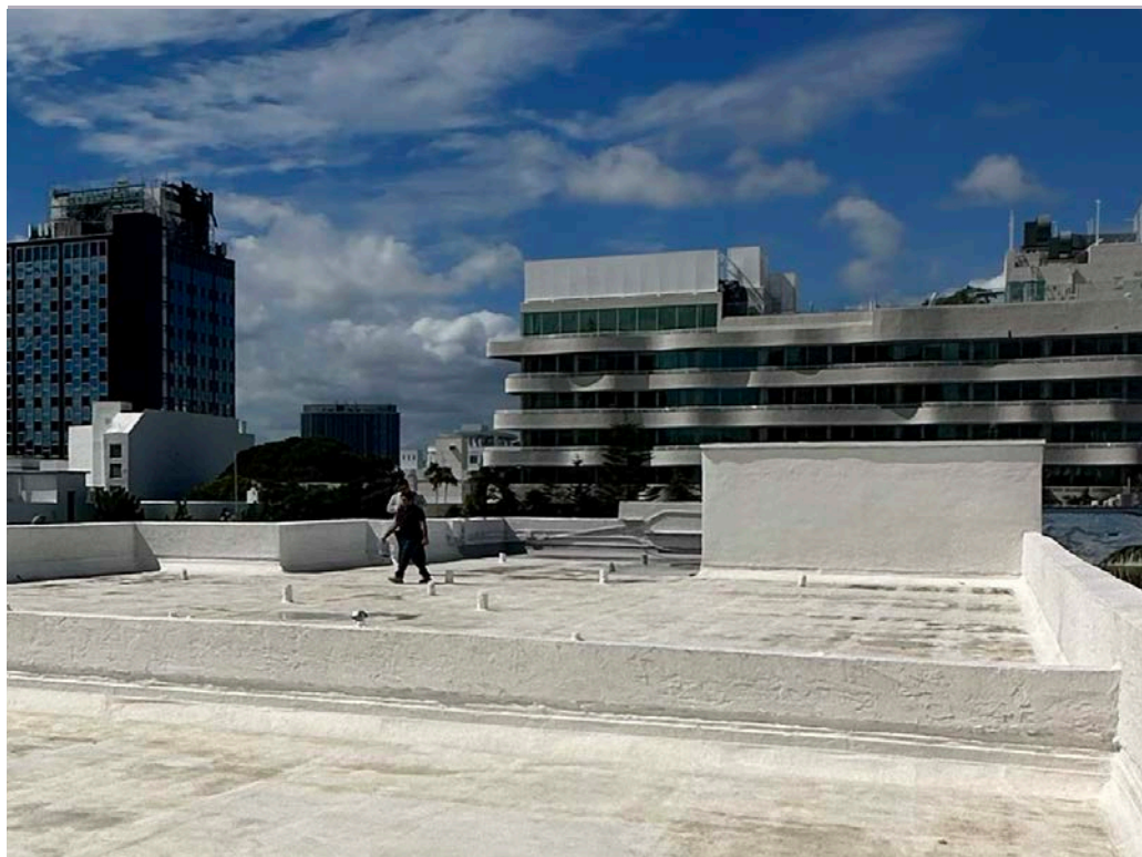
Roof level - stair
