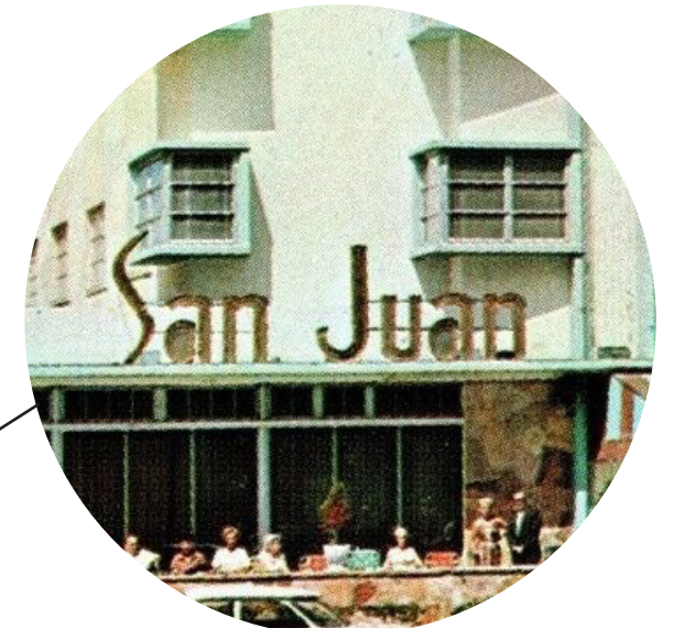
RELOCATING AND RESTORING OF HISTORIC CHANNEL LETTERS - ILLUMINATED EYEBROW MOUNTED SIGN 29'-10" W X 5'-6" H - AREA = 164 SF
