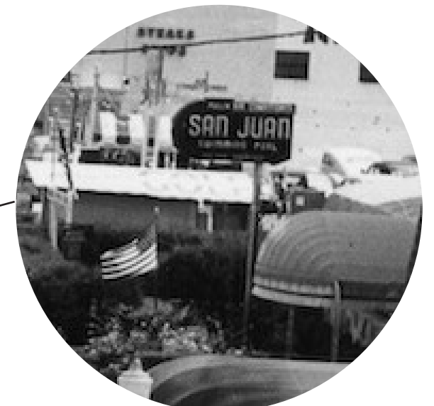
RESTORING OF HISTORIC POLE SIGN CHANNEL LETTERS - ILLUMINATED 13 FT HEIGHT SIGN DIMENSIONS = 6'-3" W X 3'-5" H - AREA = 21.3 SF
