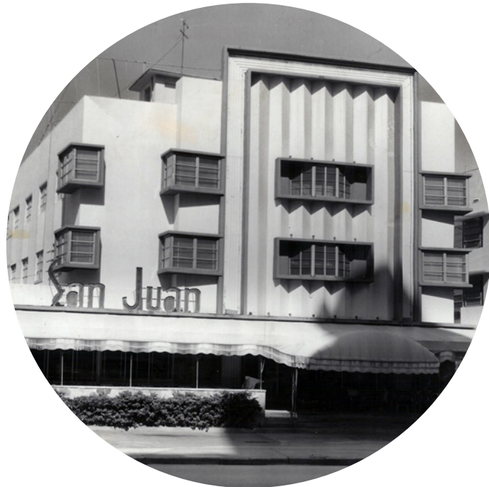
San Juan Hotel Henry Hohausner Architects 1948
