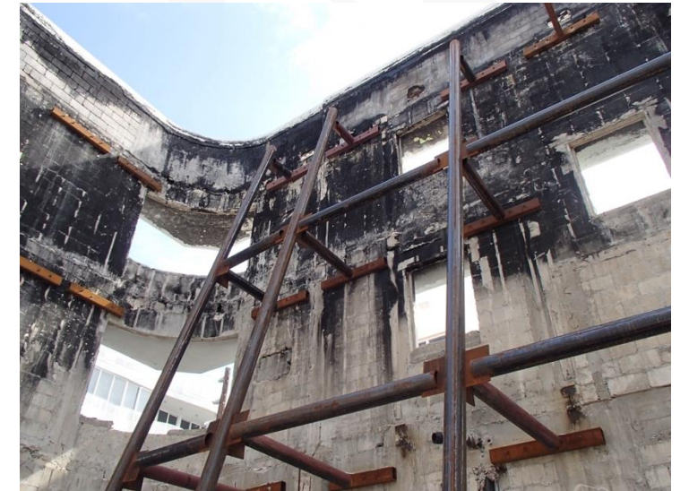
Collins Park Bracing
