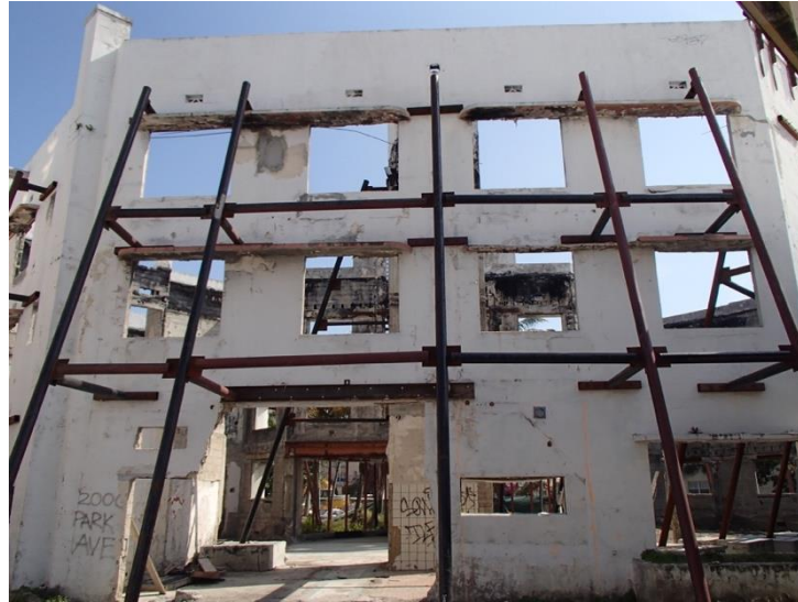
Collins Park Bracing
