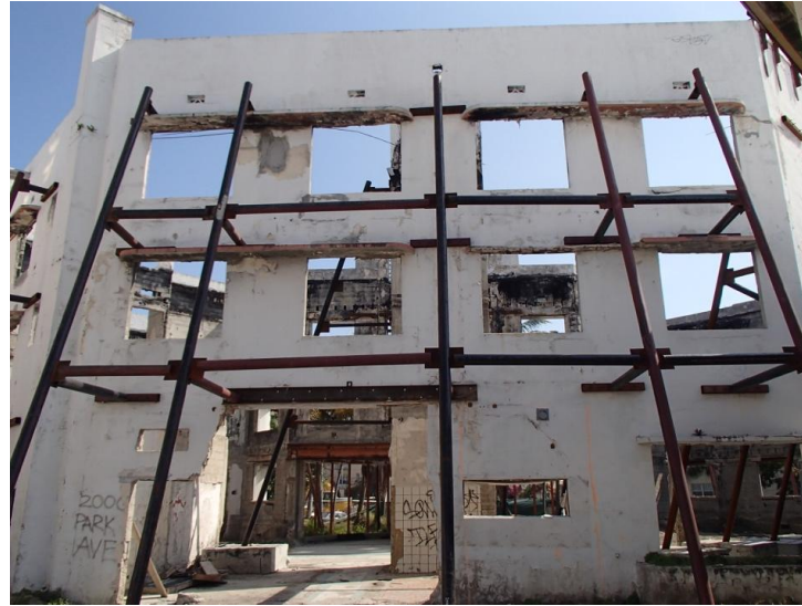
Collins Park Bracing
