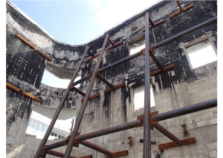
Collins Park Bracing
