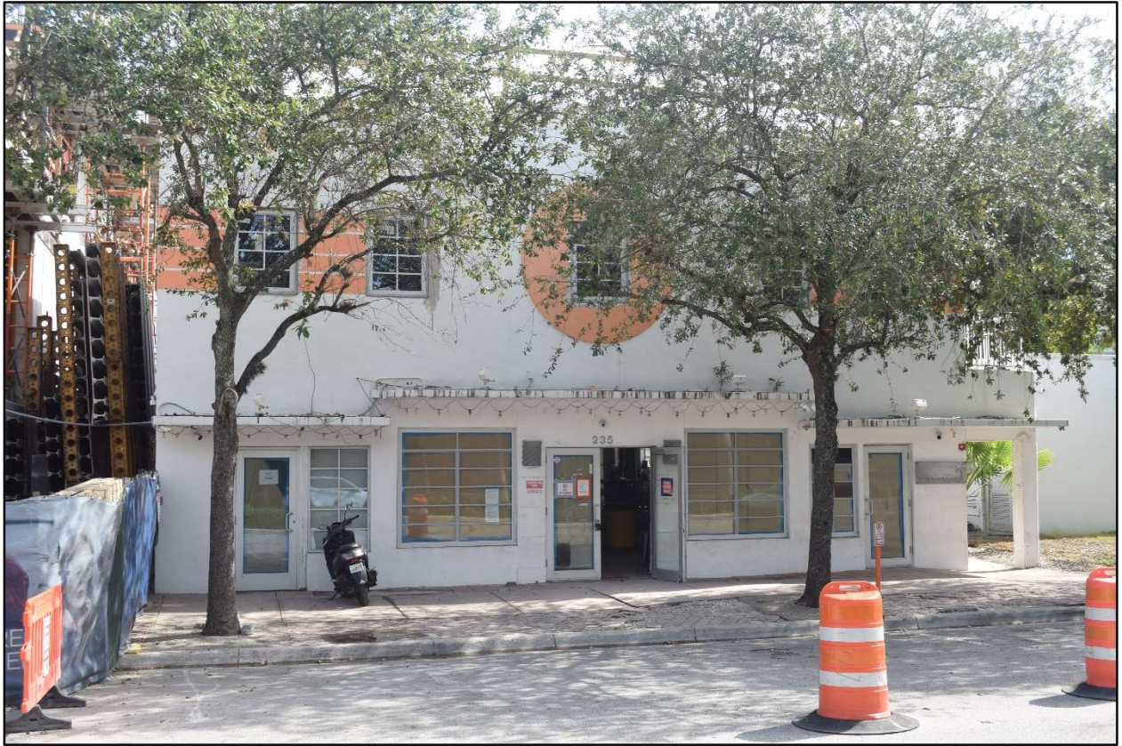
Figure 1. Former Parkside Hotel, 235 Washington Avenue, November 2025.
