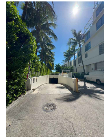
Picture #4: Subterranean tunnel
