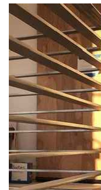
• HORIZONTAL RECTANGULAR/FLAT BAR PROFILE GUARD/HANDRAIL (ALL WELDED, NO MECHANICAL CONNECTIONS)
