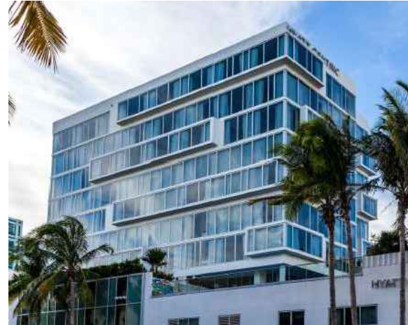
1600 COLLINS AVE, HYATT CENTRIC SOUTH BEACH EXISTING TEN STORY GLASS TOWER
