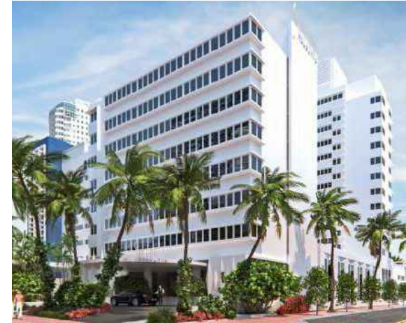
1801 COLLINS AVENUE SHELBORNE SOUTH BEACH HOTEL EXISTING EIGHT STORY ART-DECO BUILDING
