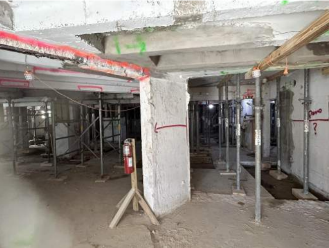
1012 Demolition Basement/Foundation Slab-on-Grade & Beam
