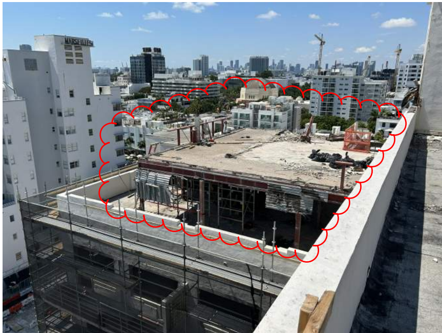
View of 8th Floor over-build Demolition
