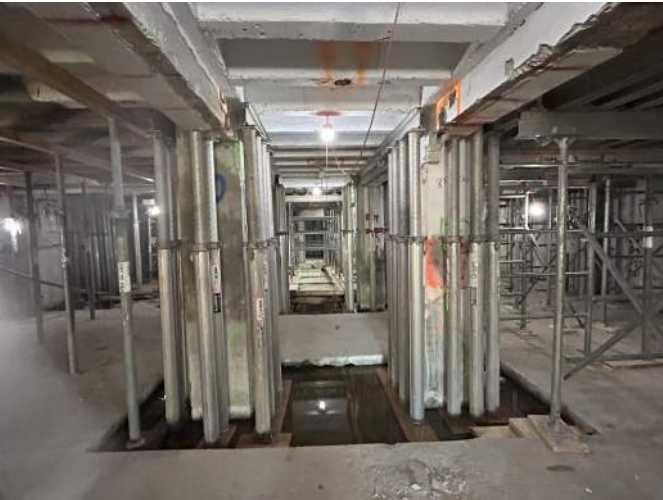
1012 Demolition Basement/Foundation Slab-on-Grade & Beam
