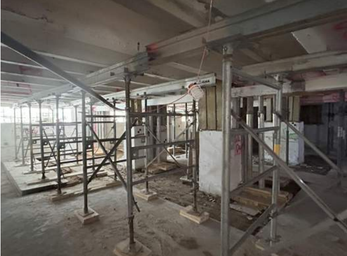
1019 Shoring at Basement
