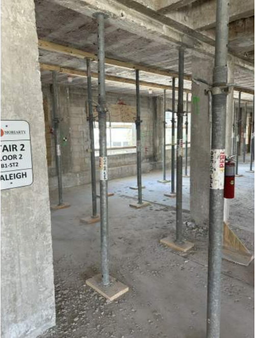
1022 Shoring at L2
