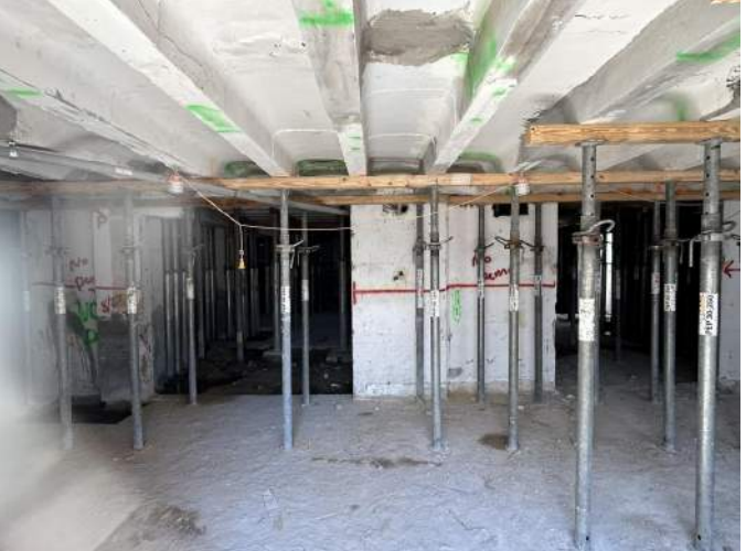
1019 Shoring at Basement
