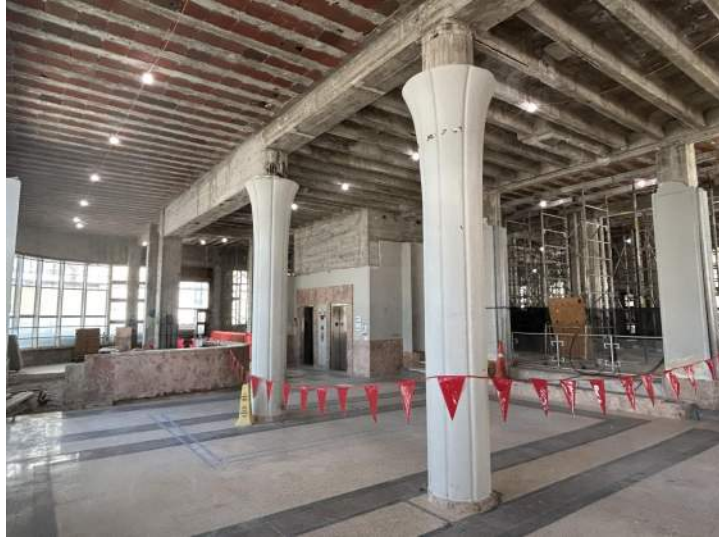
West side of lobby, currently has no shoring and/or bracing.
