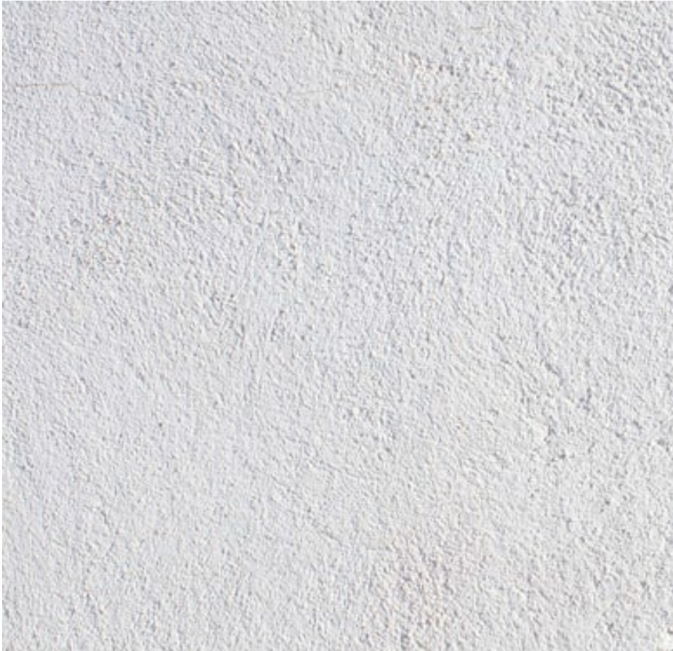
STUCCO OVER CMU
