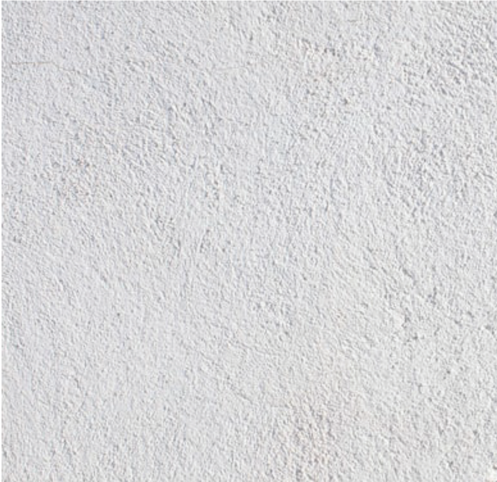
STUCCO OVER CMU
