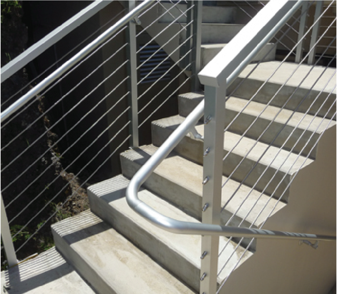
ALUMINUM GUARDRAIL
