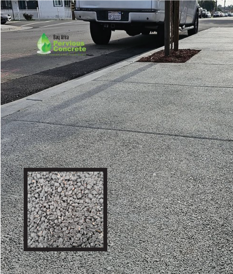
PERMEABLE CONCRETE
