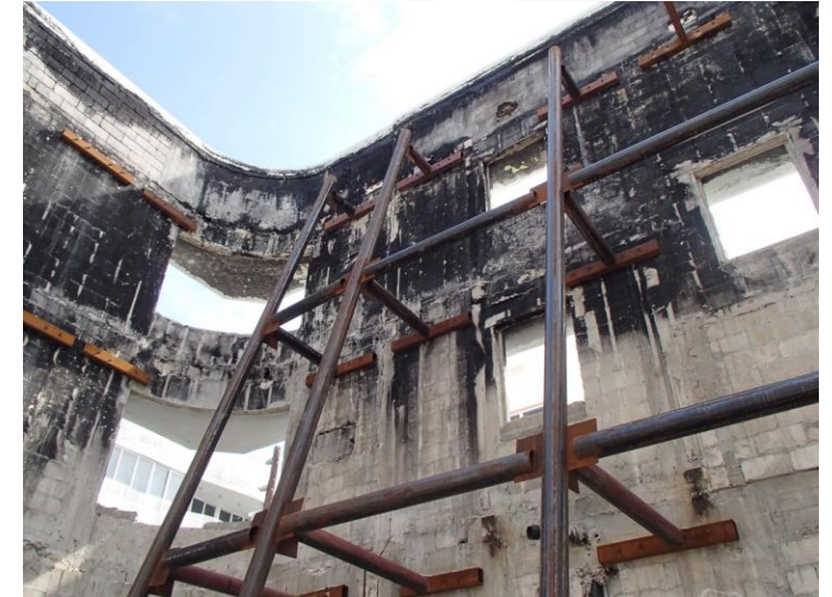
Collins Park Bracing
