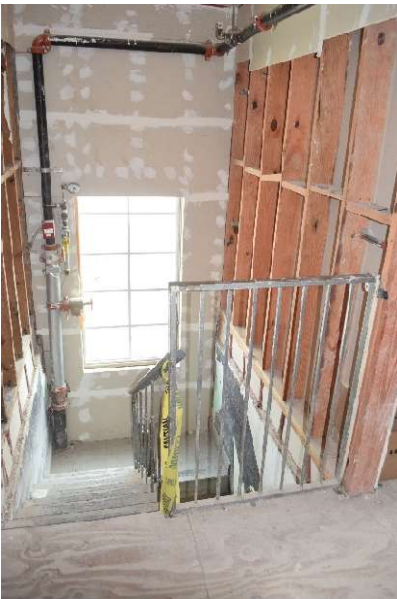
Figure 74. View of top of rear stair, looking east, November 2025.
