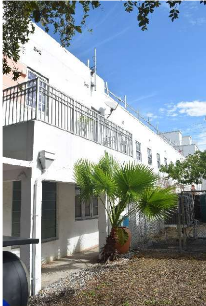
Figure 48. View of south elevation, looking northeast, November 2025.
