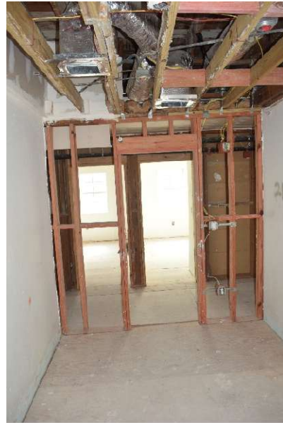
Figure 73. View of partially completed guest room, looking south, November 2025.
