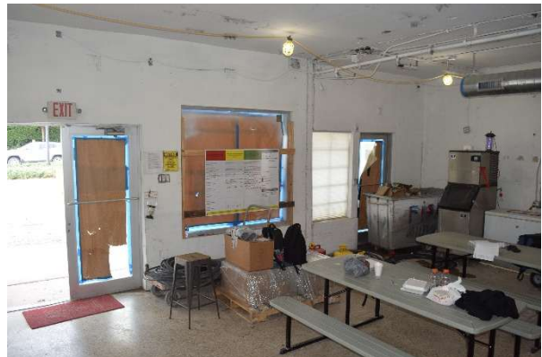
Figure 53. View of former Lobby and Mercantile space, looking northwest, November 2025.
