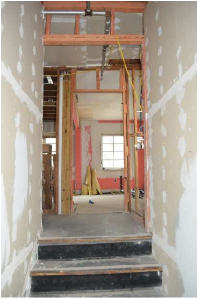
Figure 68. View of side corridor and room at top of front stairs, looking west, November 2025.
