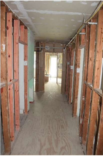
Figure 69. View of side corridor leading to upper terrace, looking south, November 2025.
