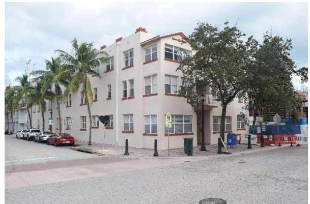
Figure 11. View of apartment building at southeast corner of Washington Avenue and 3 rd Street, looking southeast, November 2025.
