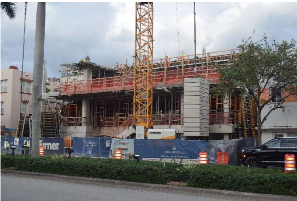
Figure 10. View of construction site at 251 Washington Avenue, looking northeast, November 2025.
