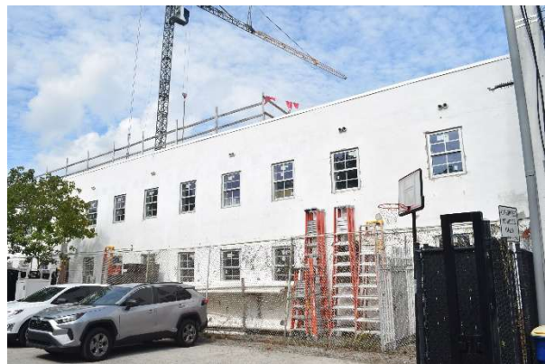
Figure 47. View of South Elevation, looking northwest, November 2025.
