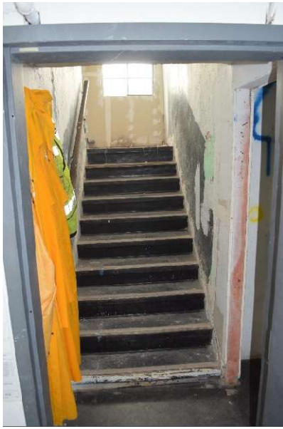
Figure 60. Detail of front stairs to Second Level, November 2025.
