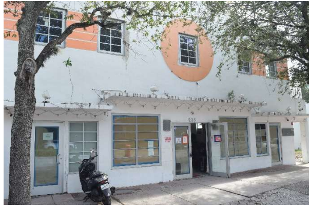
Figure 41. Detail of fenestration at Front Façade, November 2025.
