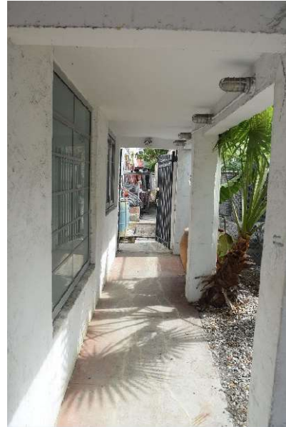
Figure 49. Detail of area under covered walkway, November 2025.
