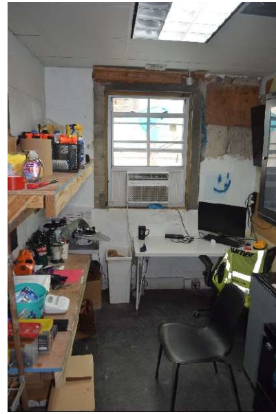
Figure 61. Detail of office adjacent front stairs, November 2025.
