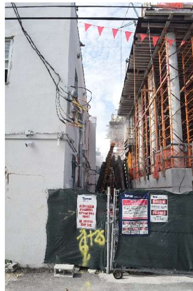
Figure 36. View of north side of site, looking west, November 2025.
