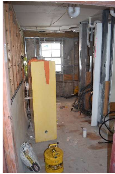
Figure 65. View of typical guest room at First Level, looking south, November 2025.
