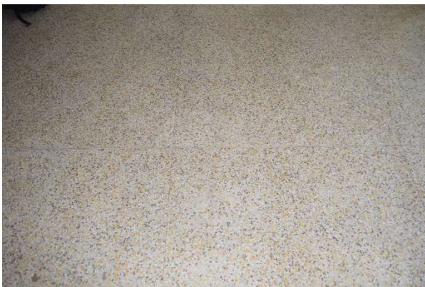
Figure 58. Detail of original terrazzo flooring, November 2025.
