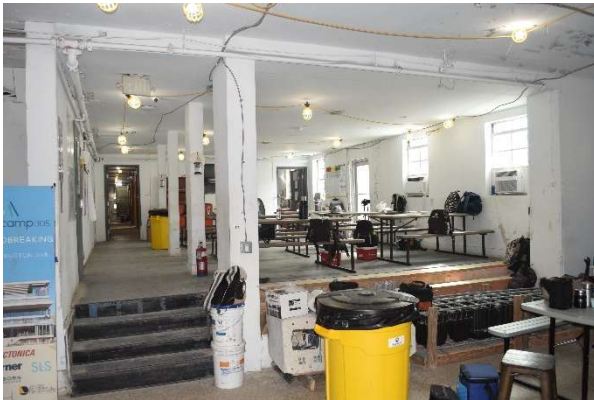
Figure 50. View of former Lobby/Check in space, looking east, November 2025.
