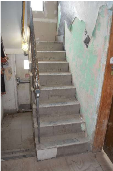
Figure 66. View of rear stairs, looking east, November 2025.
