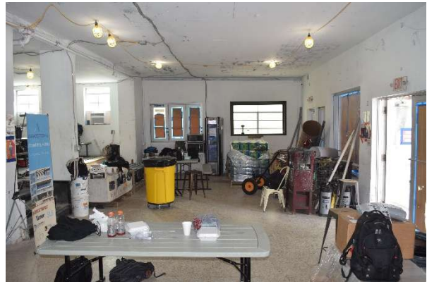
Figure 51. View of former Lobby, looking south, November 2025.
