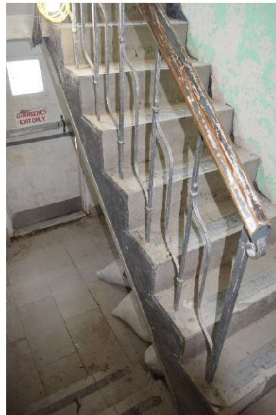
Figure 67. Detail of original balustrade at rear stairs, November 2025.
