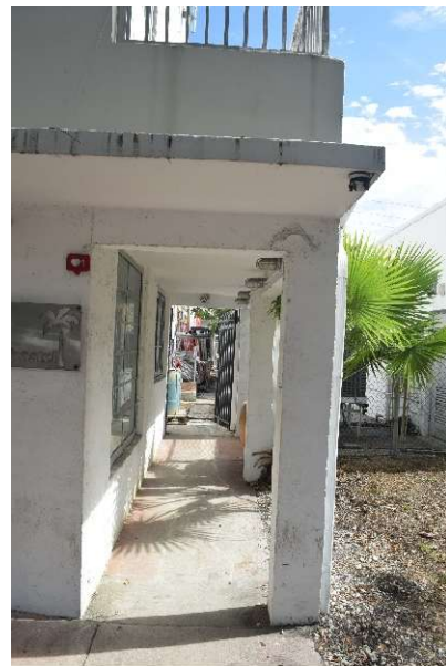
Figure 43. Detail of entrance to covered walkway, November 2025.
