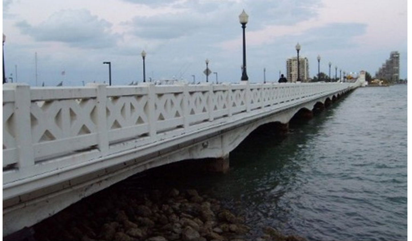
Existing Light Poles on Bridge 11
