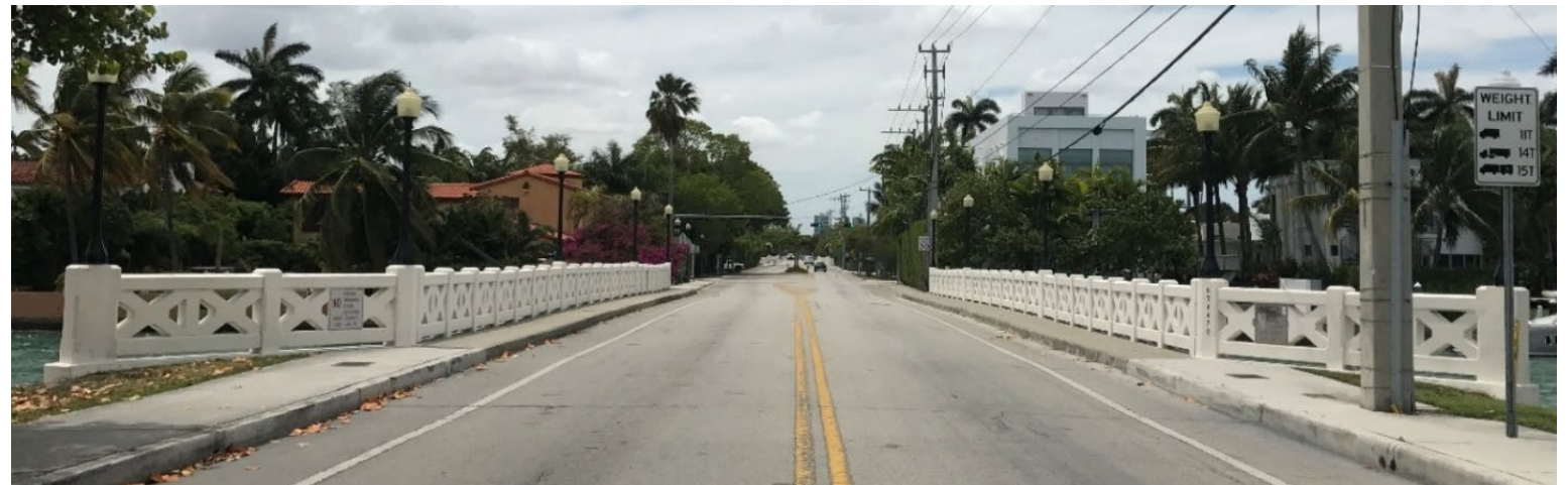
Railing on Bridge 9 from April 21, 2017
