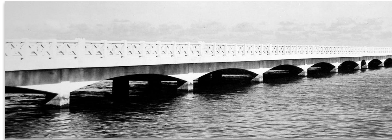
Historic Photo of Railing c. 1930s
