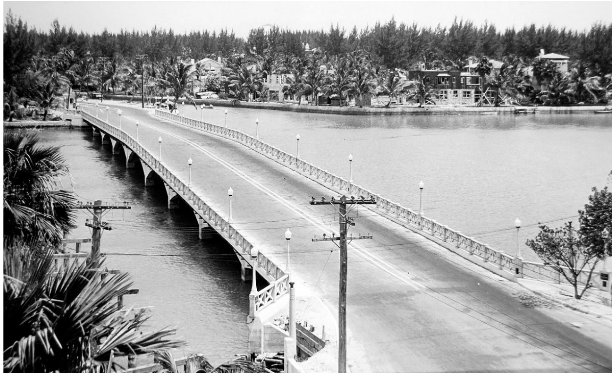
Historic Photo of Bridge 12 c. 1930s
