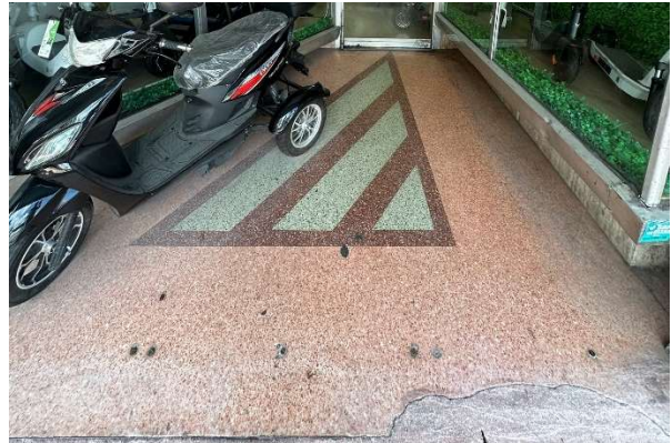
Figure 67. Detail of terrazzo floor at entrance to 1513 Washington Avenue, August 2023.
