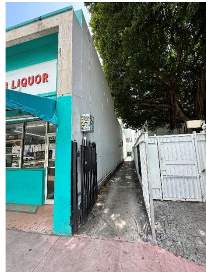
Figure 68. View of south elevation, looking east, August 2023.
