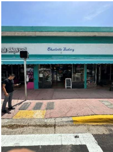
Figure 44. View of 1499 Washington Avenue, August 2023.
