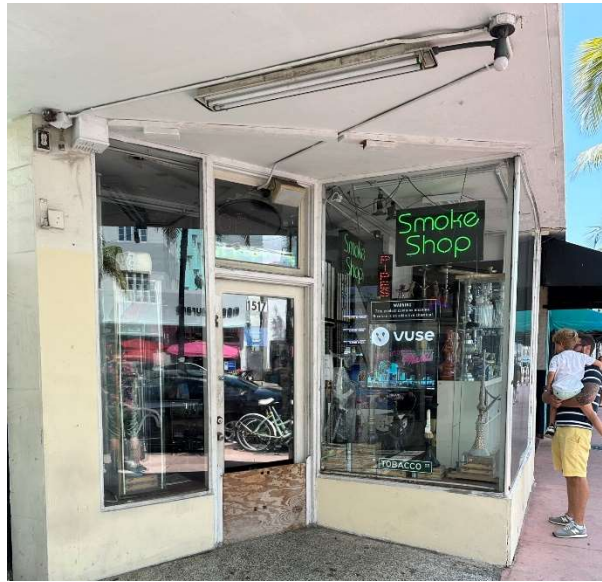
Figure 79. Detail of entrance to 1517 Washington Avenue, August 2023.
