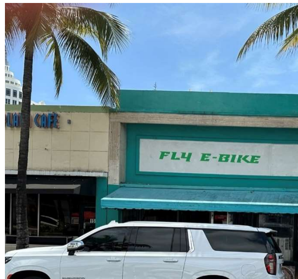
Figure 37. Detail of north end of building that abuts neighboring building, August 2023.
