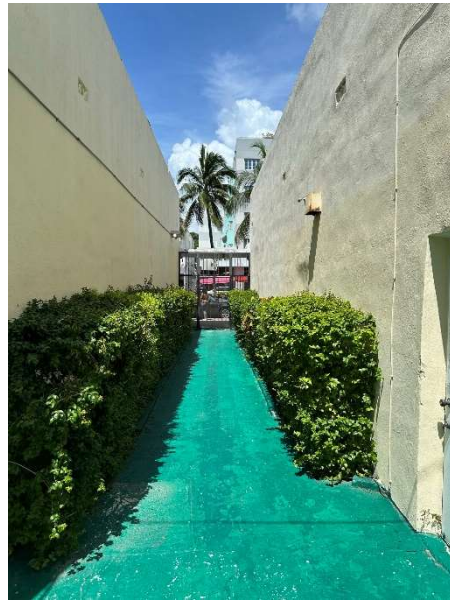
Figure 86. View of walkway to rear building, looking west, August 2023.
