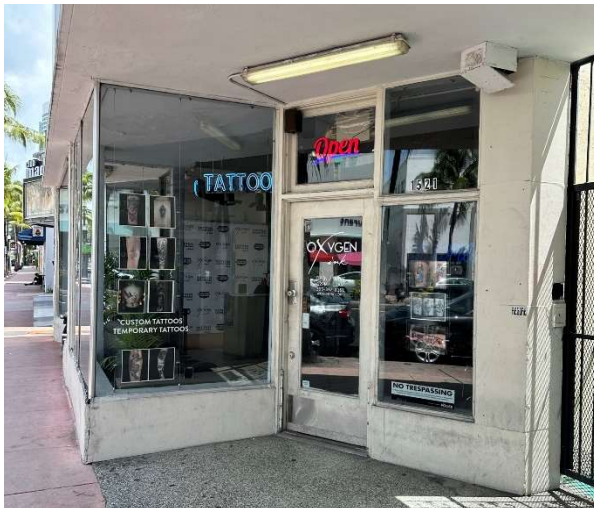
Figure 81. Detail of entrance to 1521 Washington Avenue, August 2023.
