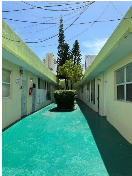
Figure 92. View of courtyard at interior of “U” at rear building, looking east, August 2023.
