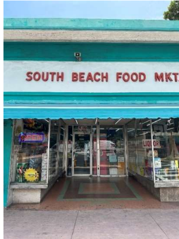
Figure 42. View of 1493 Washington Avenue, August 2023.
