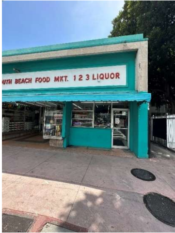
Figure 41. View of 1491 Washington Avenue, August 2023.
