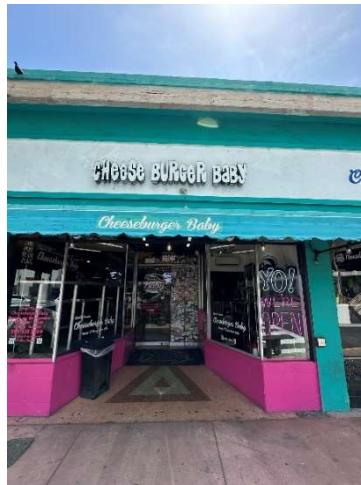
Figure 45. View of 1505 Washington Avenue, August 2023.
