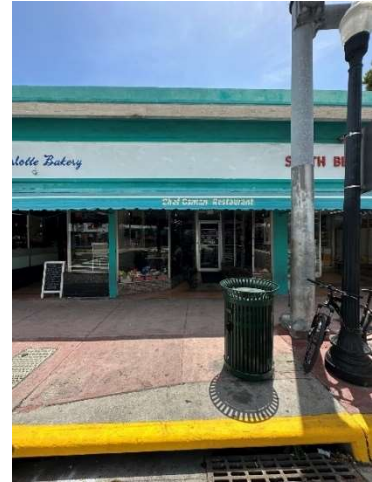
Figure 43. View of 1497 Washington Avenue, August 2023.
