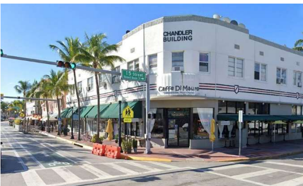
Figure 14. View of west side of Washington Avenue, looking south from 15 th Street, February 2021. (Google Earth)
