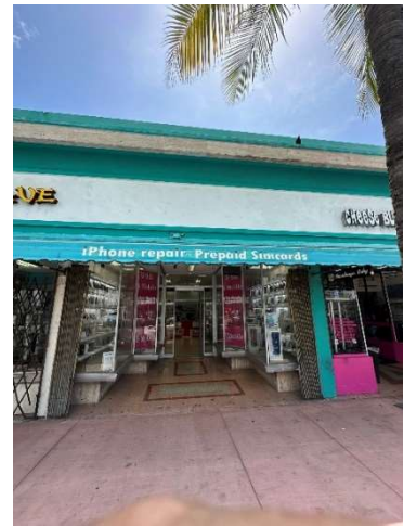
Figure 46. View of 1507 Washington Avenue, August 2023.
