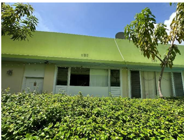
Figure 95. View of Unit 3, looking south, August 2023.
