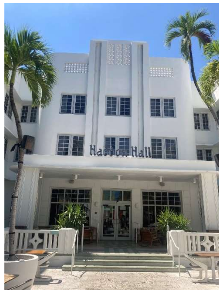
Figure 27. View of central bay, September 2023.
