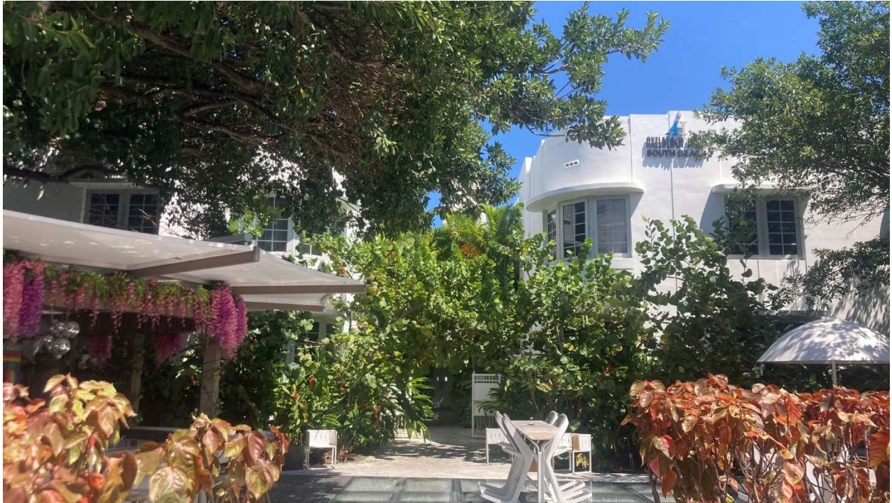
Figure 2. 1453-55 Washington Avenue, September 2023.
