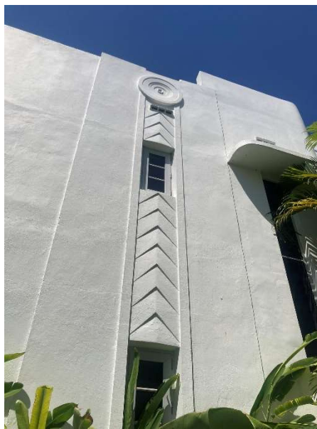
Figure 40. Detail of chevron motif and medallion, September 2023.
