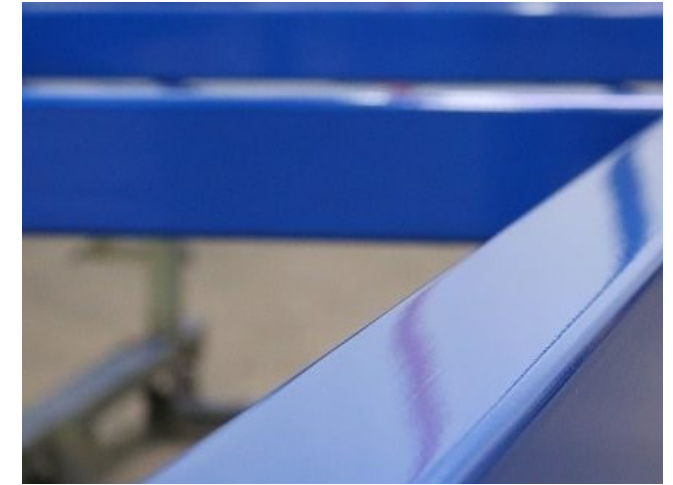
MTL-03: PAINTED BLUE, GALVANIZED, STEEL PICKET GUARDRAIL
