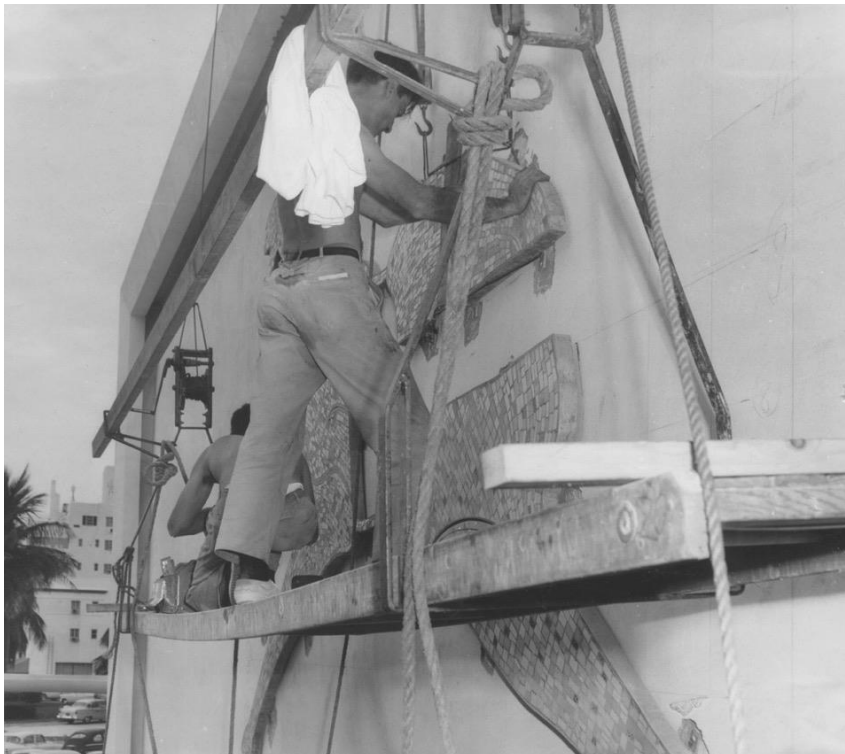
Ca. 1959 photograph of the installation of the mural on the Versailles Hotel.
