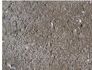
Seashell Concrete for Apparatus Bay Ramps
