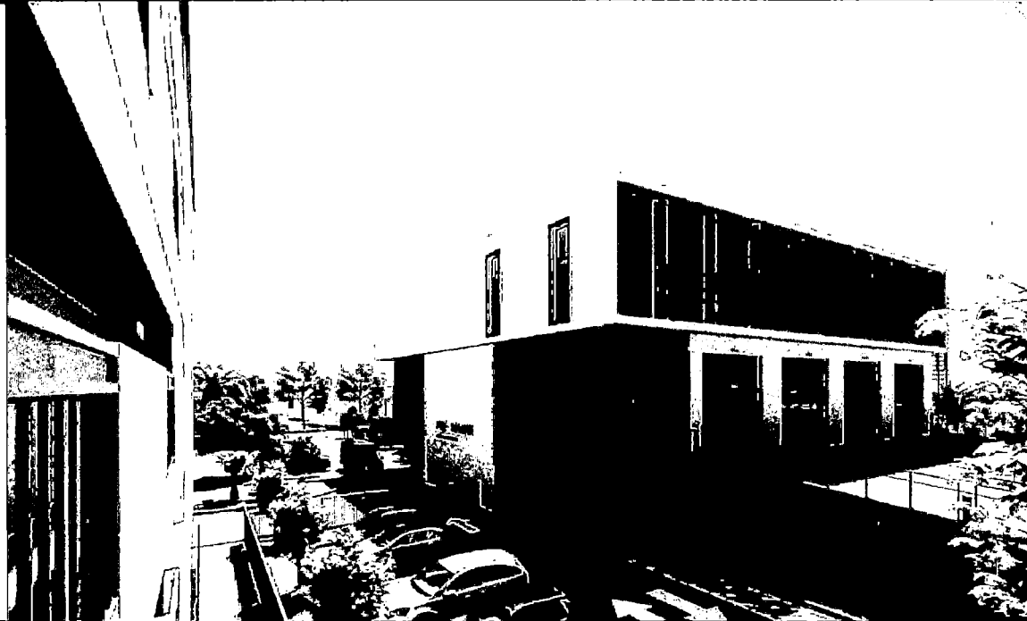
VIEW NW CORNER – NORTH ELEVATION
