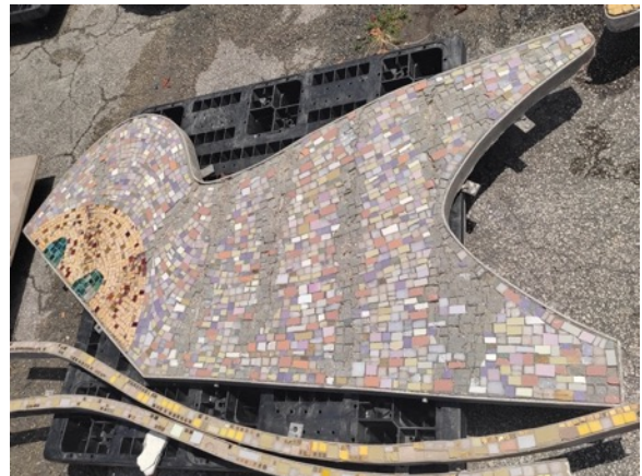
Overall of panel #20 after relocation, cleaning and removal of additional loose tiles.
