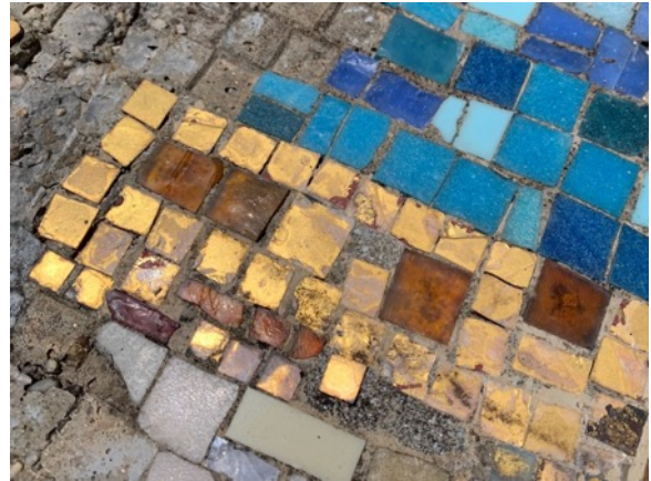
Detail of panel #1, showing translucent square amber tiles with dark/black bio growth visible between the back of the tile and the mortar bed, and gold leaf tiles where thin glass surface has been compromised and spalled, turning light pink.
