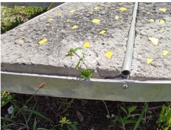
Detail of hollow, superficial aluminum decorative tube on 'ground' panel.
