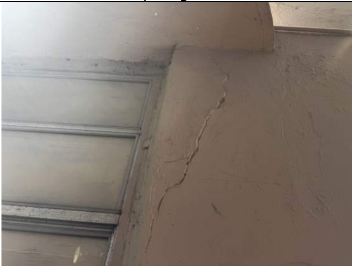
Concrete cracking
