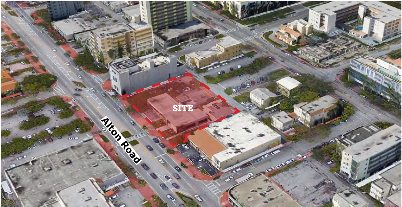
02 - EXISTING AERIAL VIEW NORTHEAST
