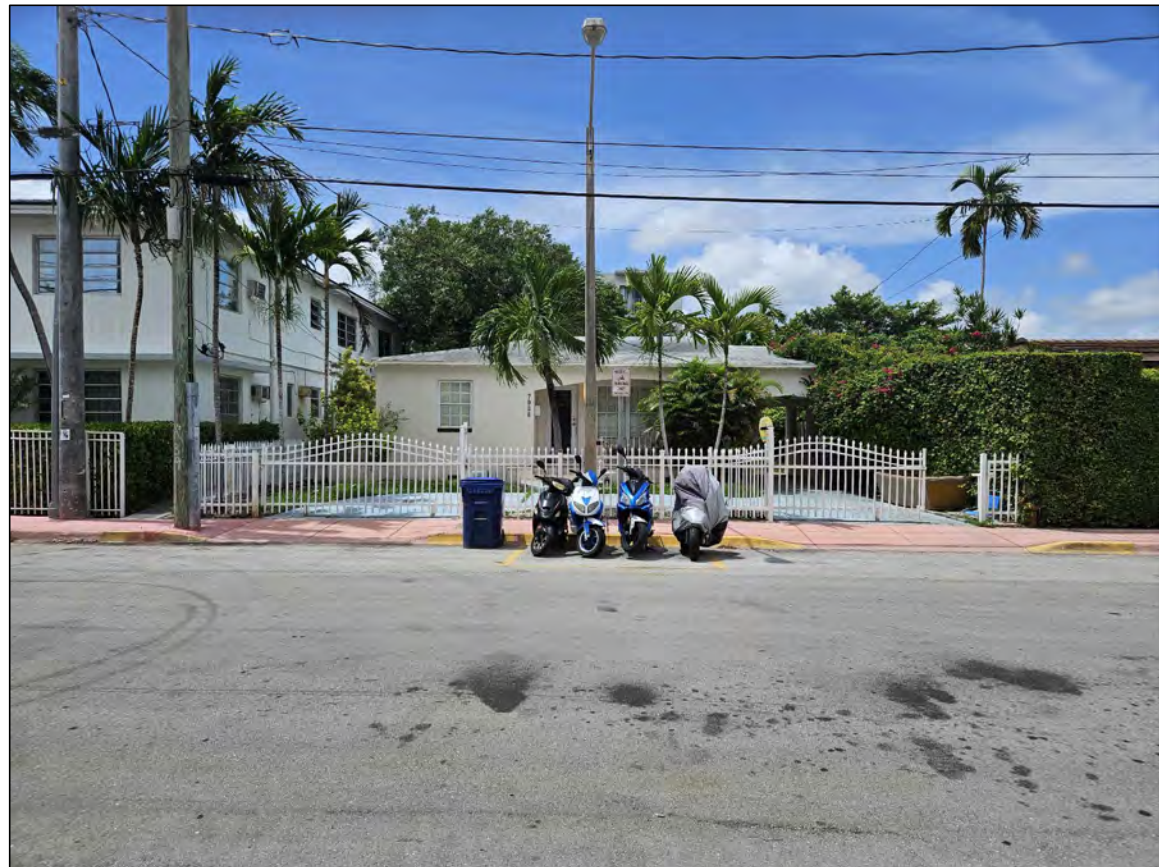
EAST FACADE - VIEW FROM OPPOSITE SIDEWALK
