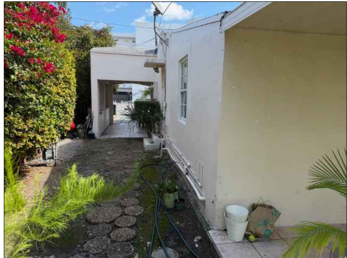
PORTE COCHERE AND NORTH FACADE - VIEW FROM REAR OF PROPERTY
