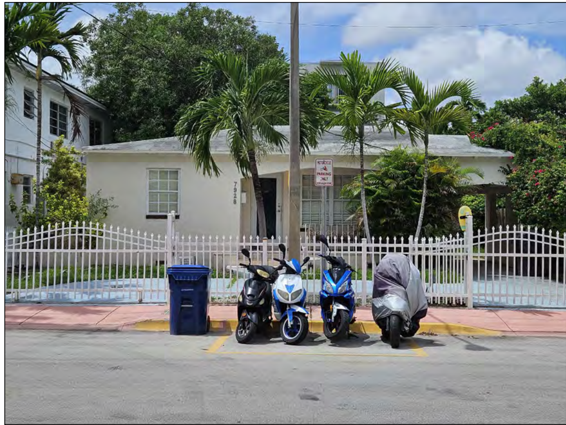
EAST (FRONT) FACADE -VIEW FROM BYRON AVENUE
