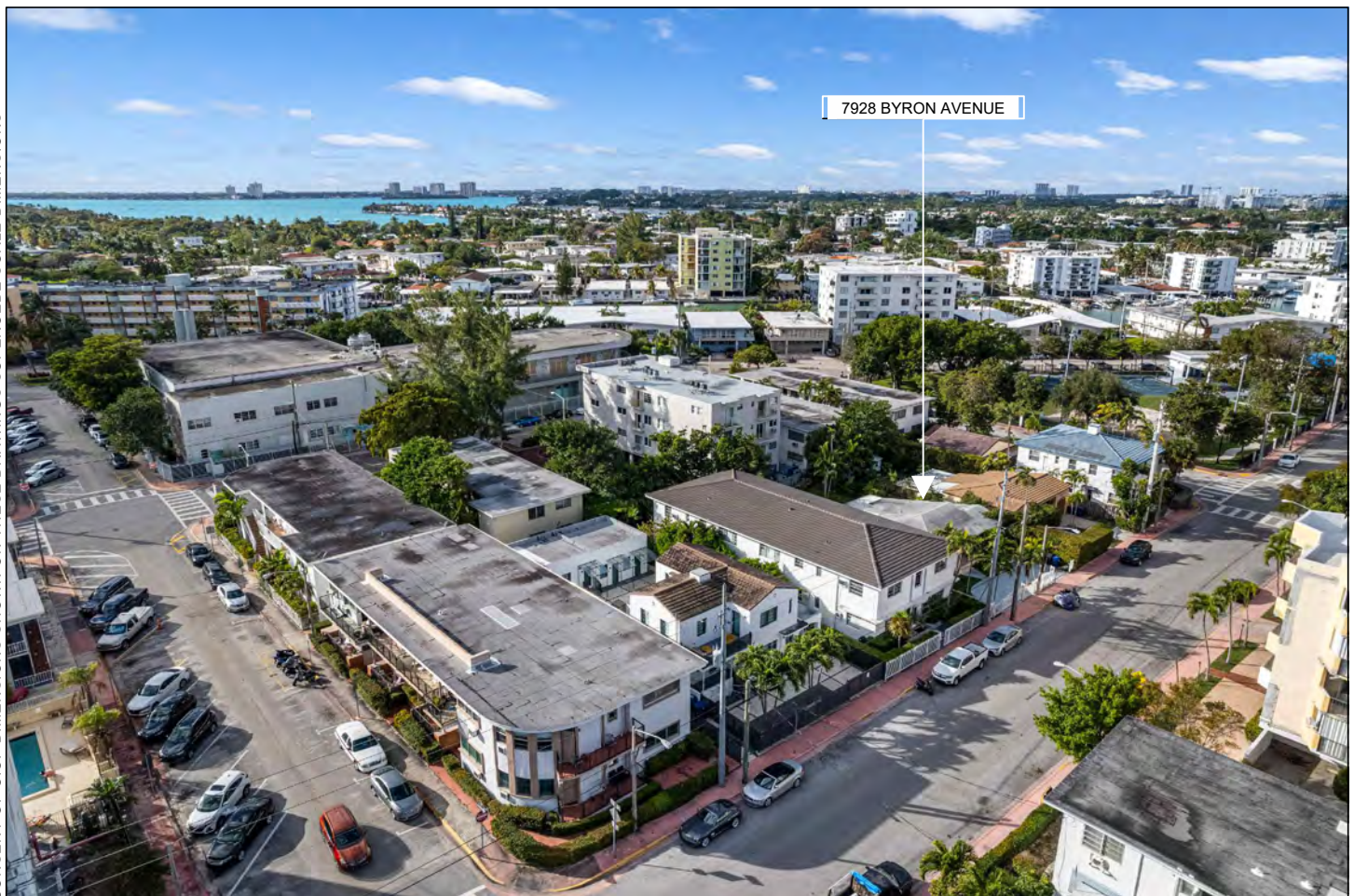
AERIAL VIEW FACING NW
