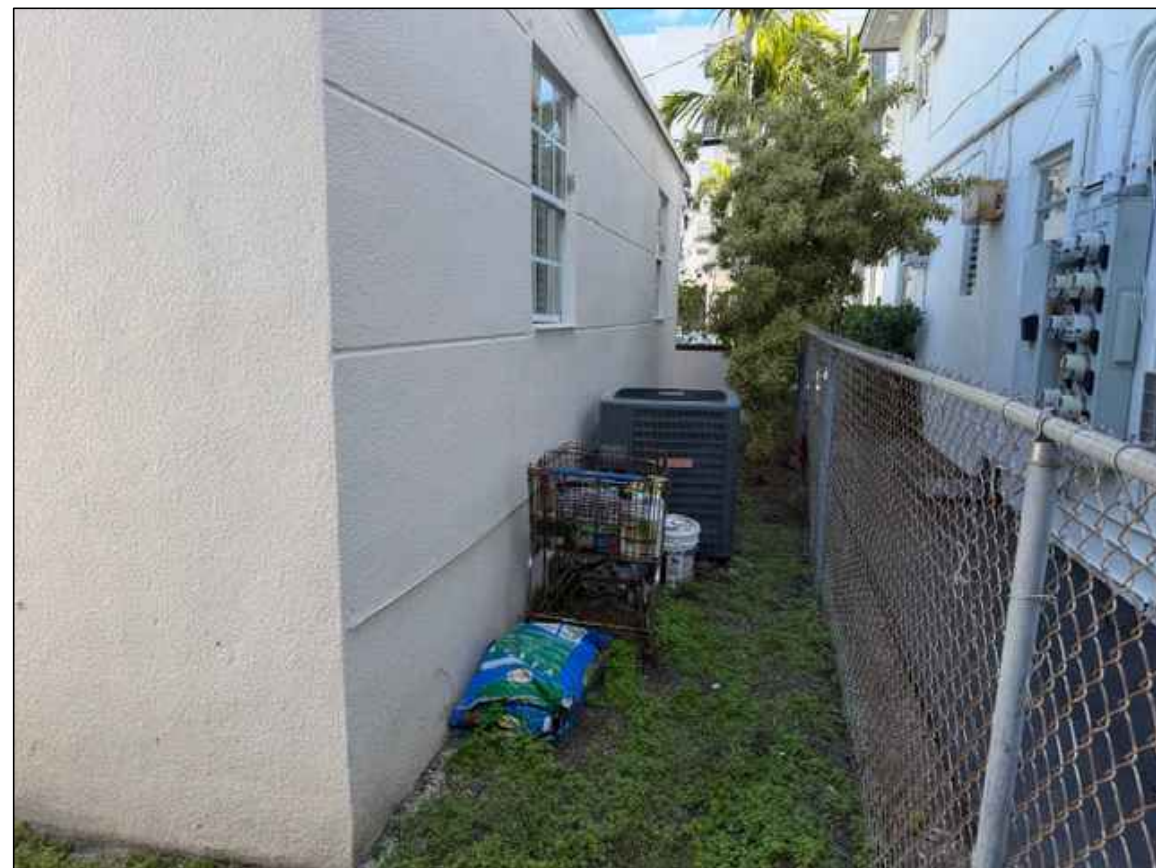
SOUTH FACADE - VIEW FROM REAR OF PROPERTY
