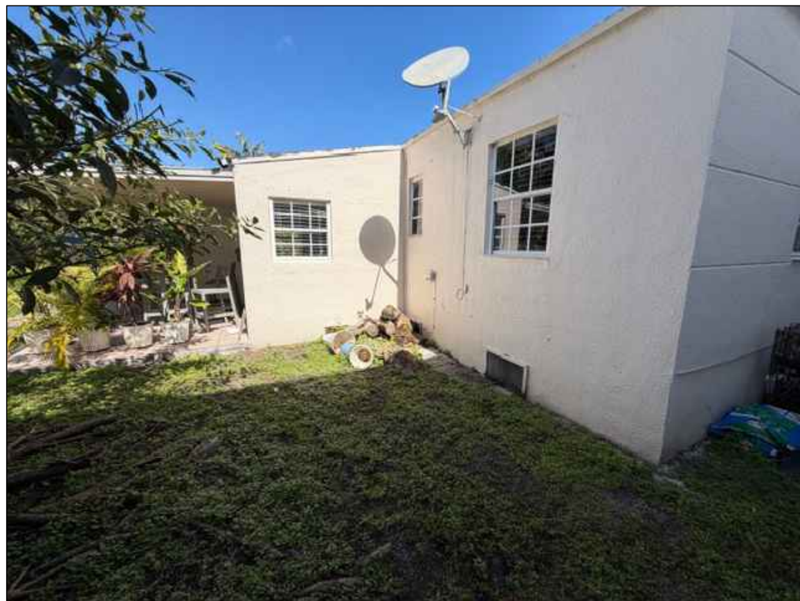
WEST (REAR) FACADE - VIEW FROM SW
