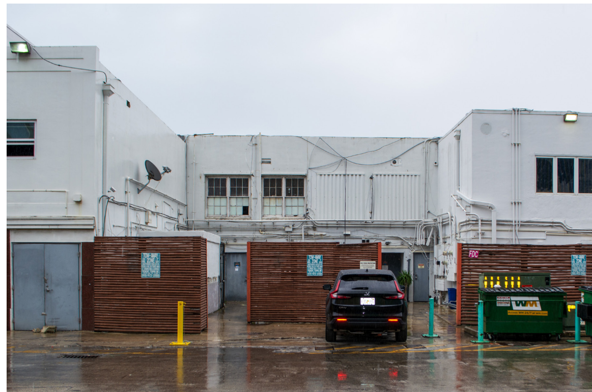
C. LINCOLN LANE (SOUTH FACADE)
