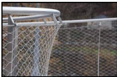
M03 ALUM. RAILING WITH MINI-MESH FABRIC
