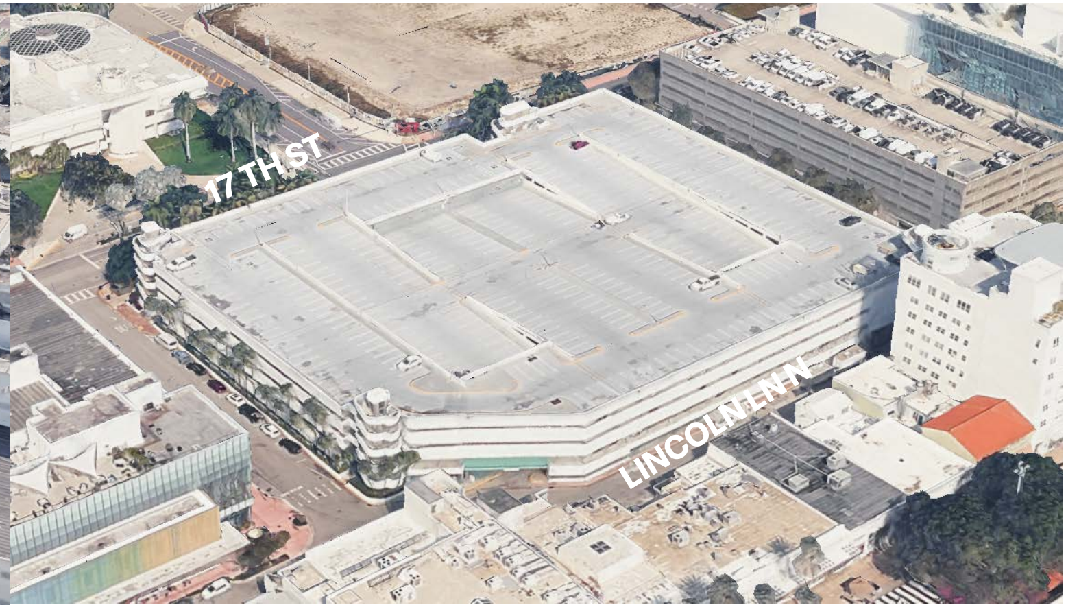
1: SW AERIAL VIEW
