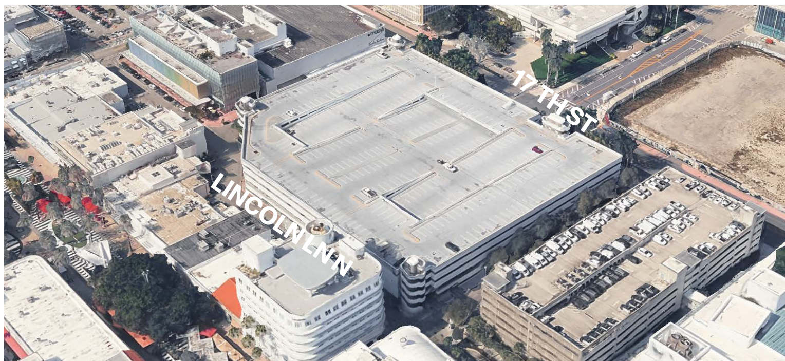
1: SE AERIAL VIEW
