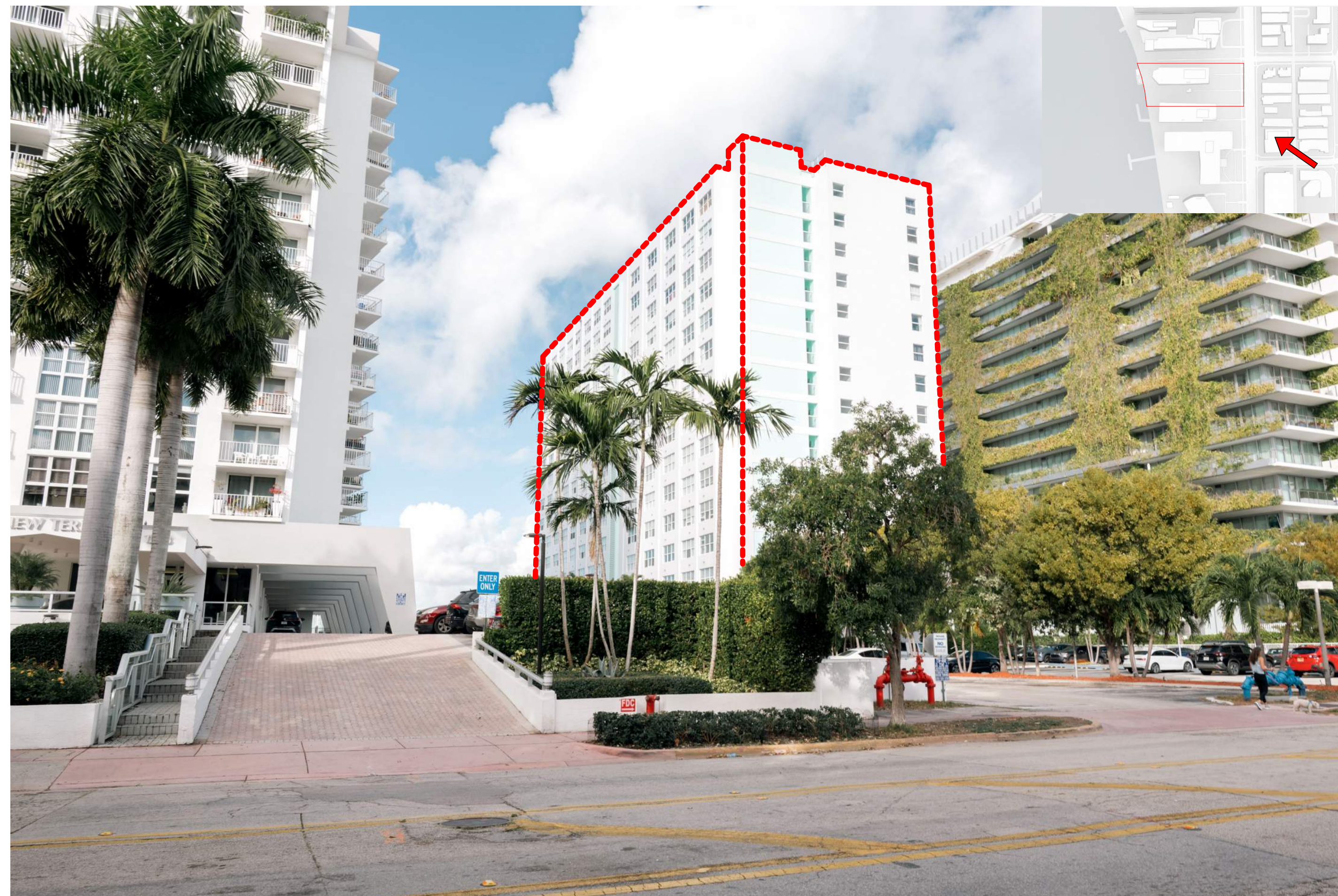
02 VIEW FROM WEST AVE
