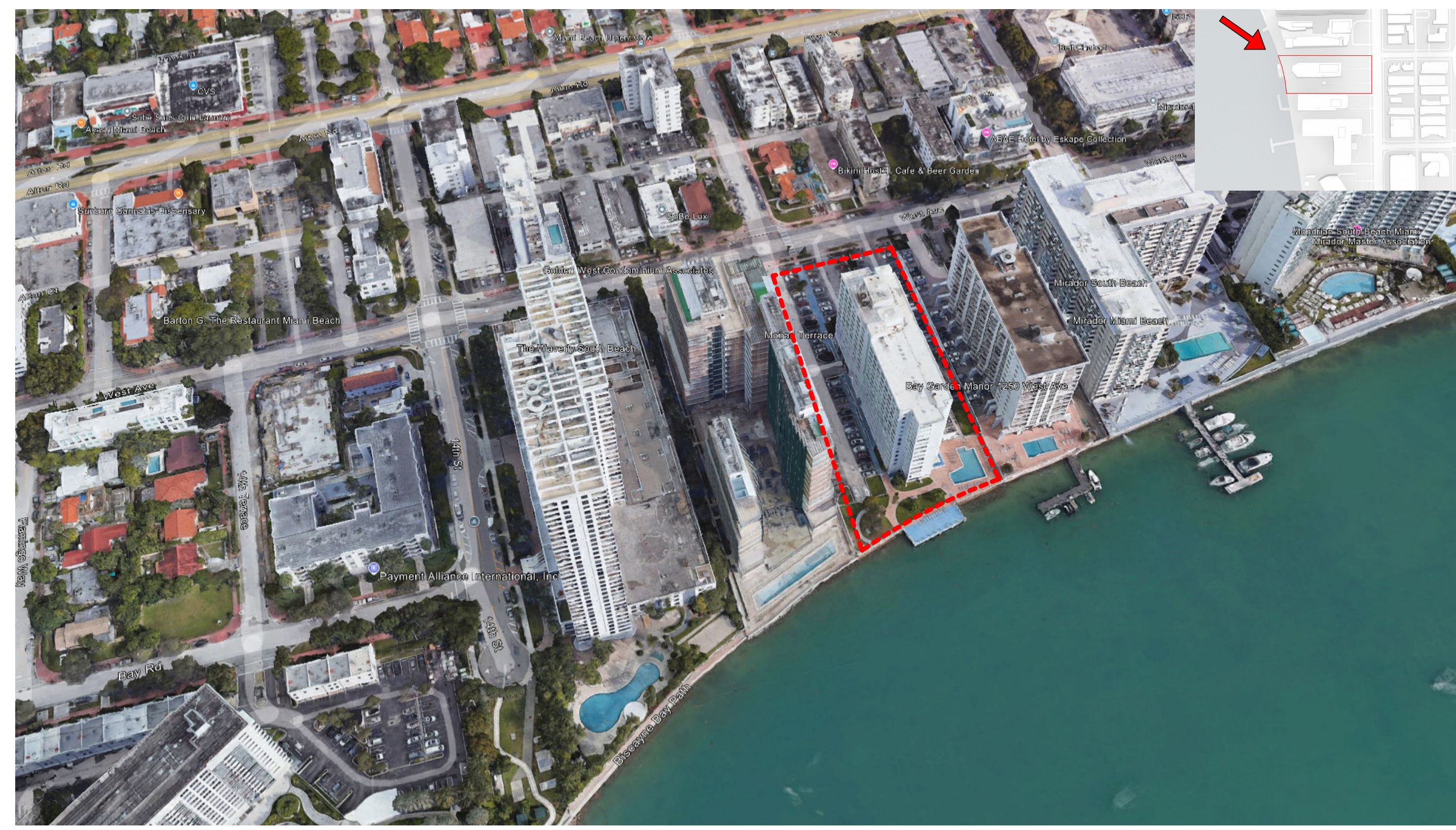
03 AERIAL VIEW - FROM NORTH
