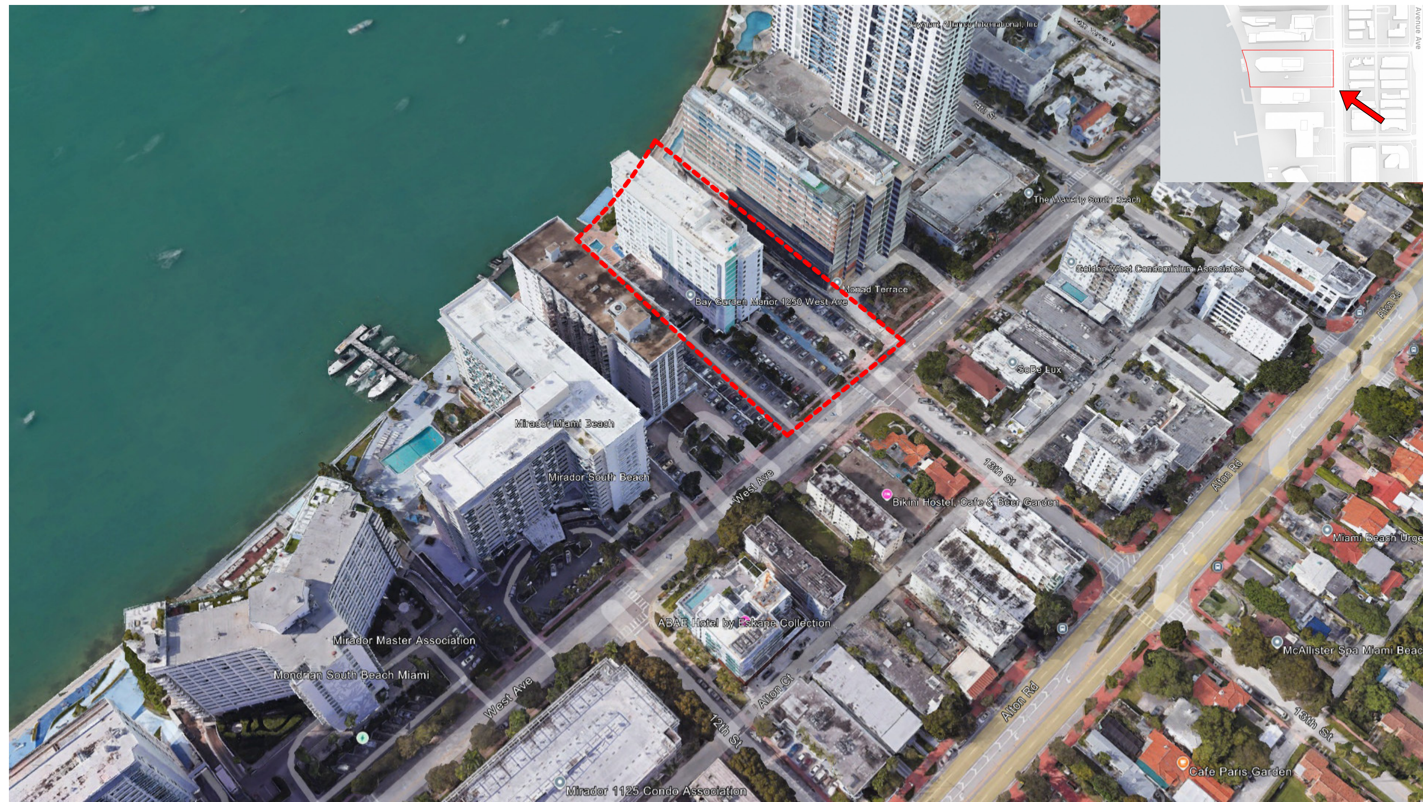
04 AERIAL VIEW - FROM NORTH
