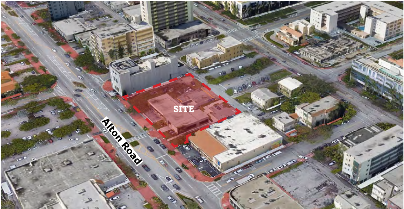
02 - EXISTING AERIAL VIEW NORTHEAST
