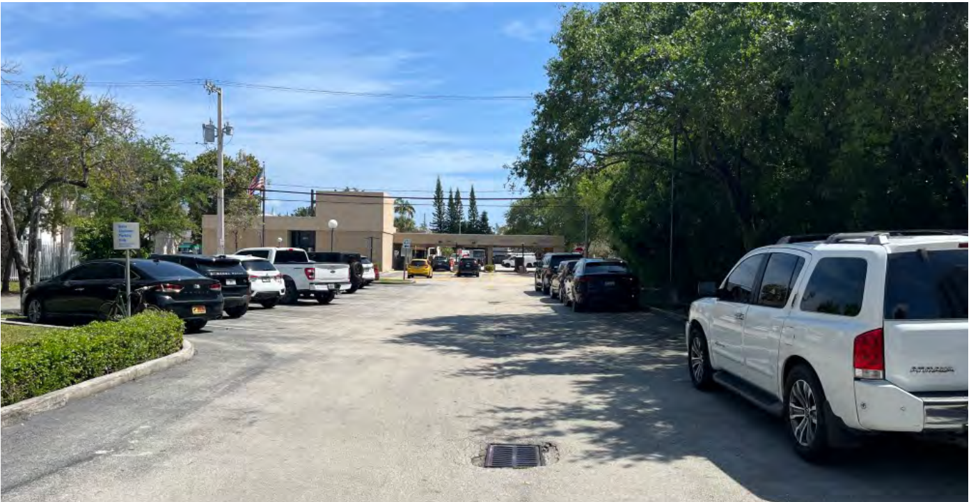
02 - VIEW OF EXISTING STRUCTURE FROM WEST AVE
