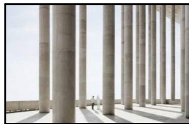
M11 PIP-CONC. COLUMN - PAINTED
