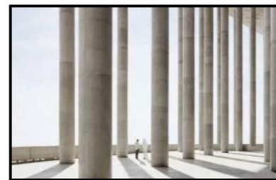
M11 PIP-CONC. COLUMN - PAINTED
